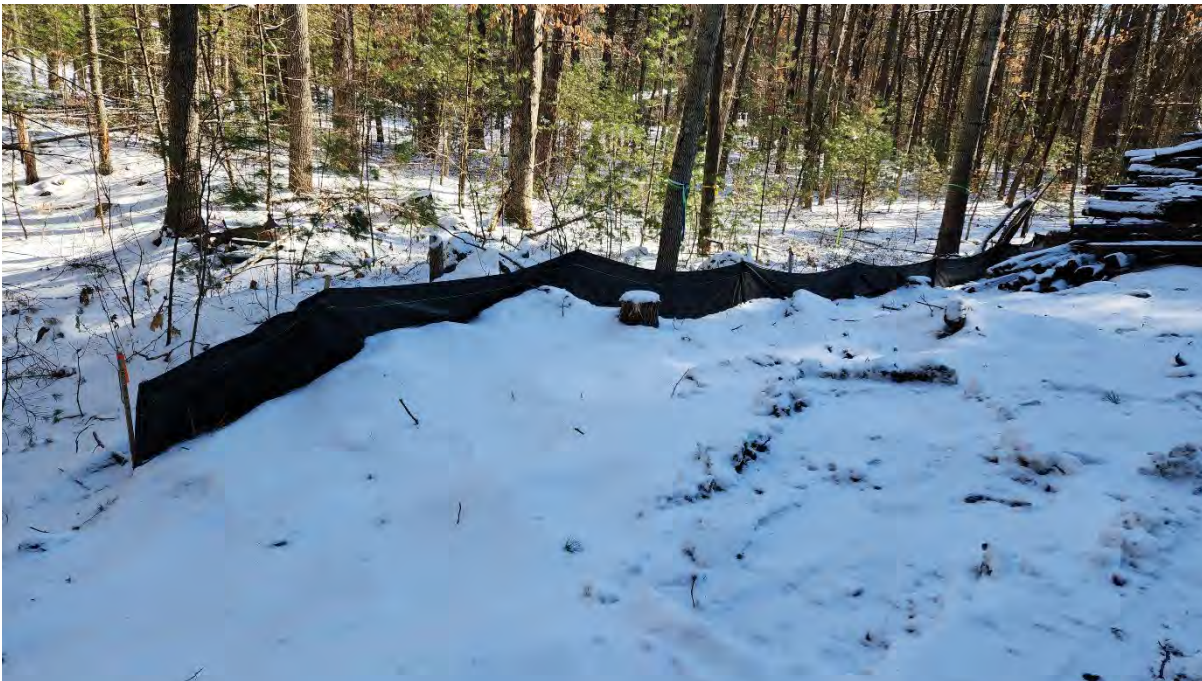
Photo 6: Silt fence installed along segment 8. Photo taken on 2/27/23
