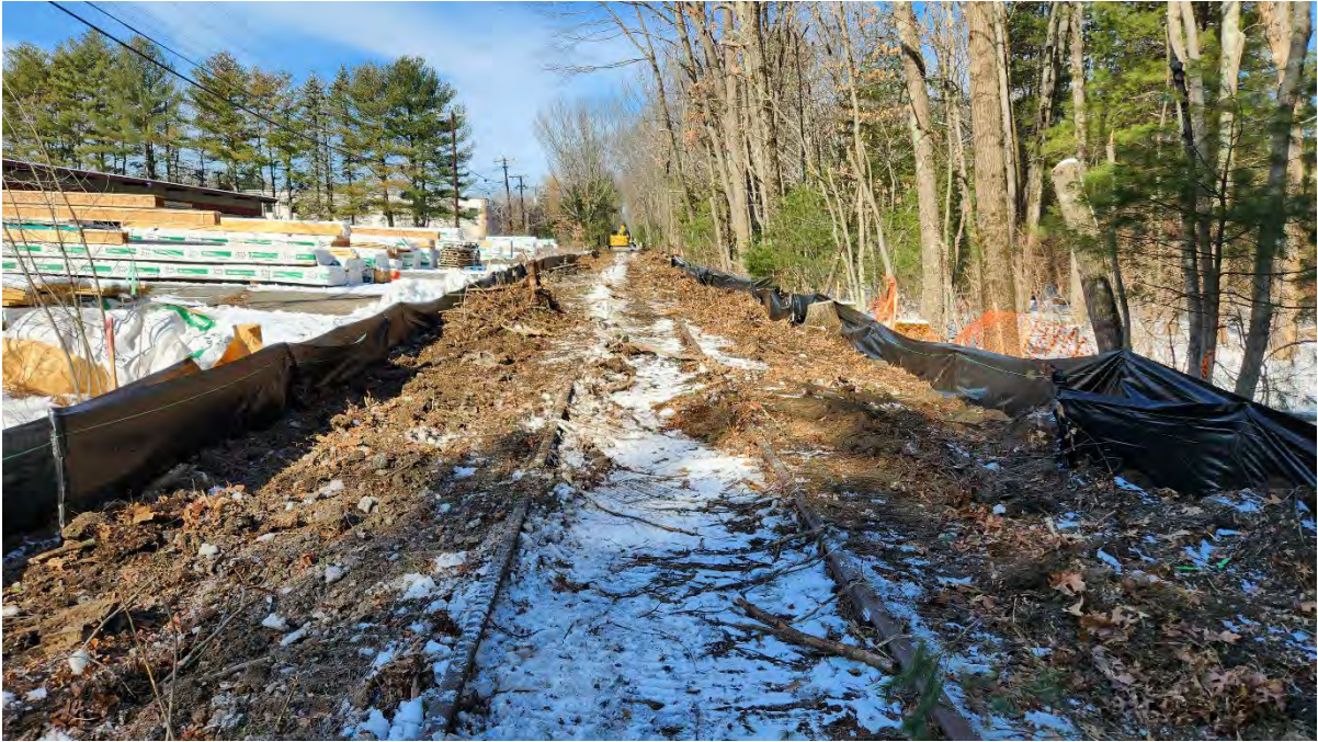
Photo 3: Silt fence installed along segment 11. Photo taken on 2/27/23
