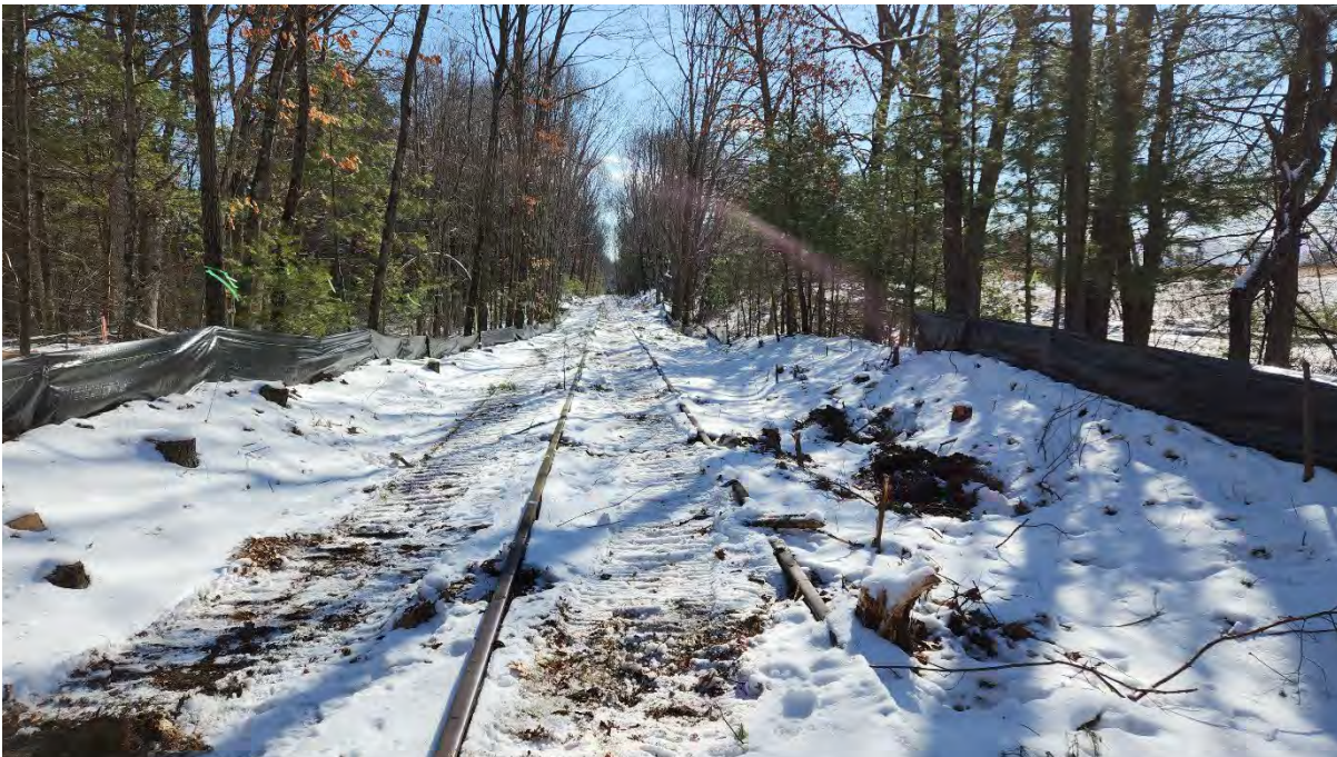
Photo 4: Silt fence installed along segment 10. Photo taken on 2/27/23
