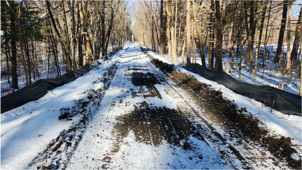
Photo 5: Silt fence installed along segment 9. Photo taken on 2/27/23
