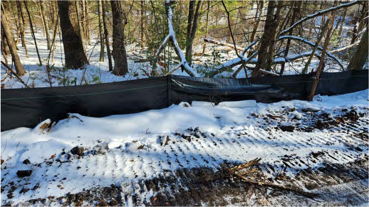
Photo 7: Silt fence installed along segment 7. Photo taken on 2/27/23
