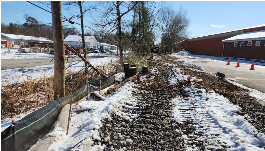
Photo 2: Silt fence and filter tube installed at Union Avenue (STA 407+50). Photo taken on 2/27/23
