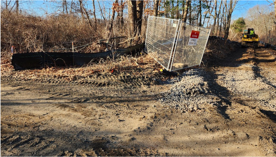
Photo 1: Silt fence at the cleared gravel site entrance (Boston Post Road, STA 476+00). Photo taken on 1/11/23
