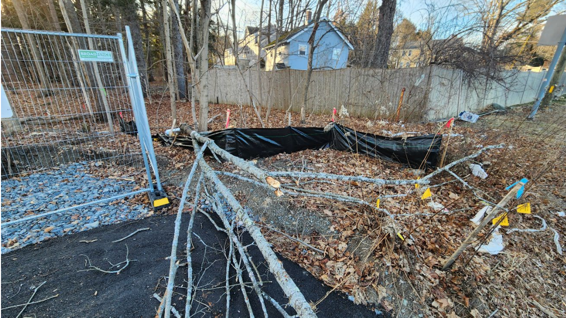
Photo 3: Gravel site entrance (Boston Post Road, STA 420+00) where a tree had fallen onto the silt fence.
