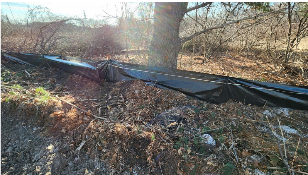
Photo 2: Silt fence installed along Segment 14.
