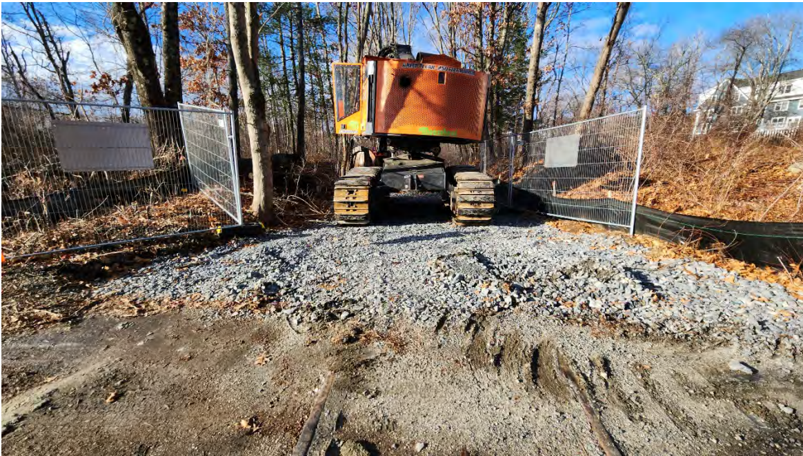
Photo 1: Feller buncher at the gravel site entrance (Boston Post Road, STA 476+00) during the beginning of tree clearing.
