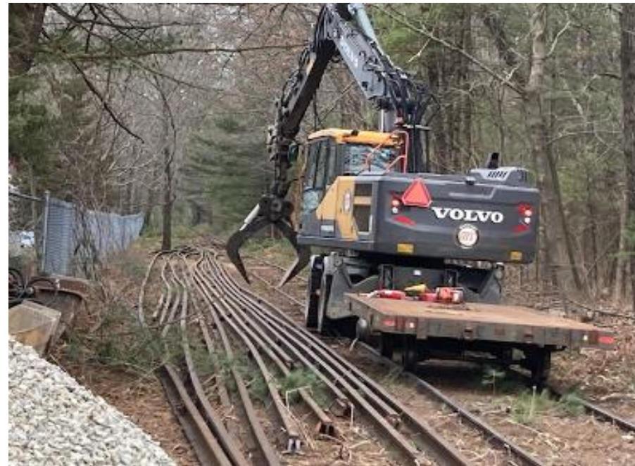
Construction Work at Hudson Road
