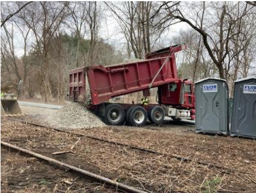
Gravel Dump at Hudson Road
