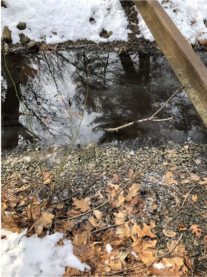
Photo 5. A portion of the Bank within limit of work is comprised of small stone and gravel and has washed into the stream
