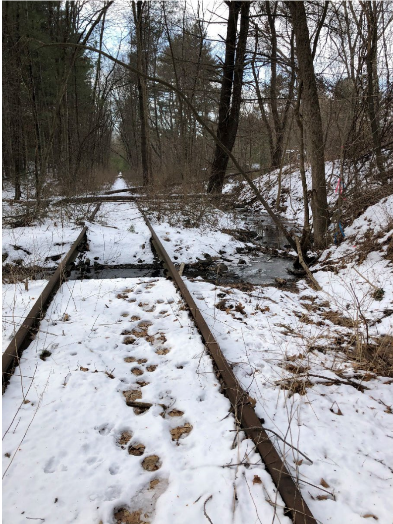
Photo 1. Existing railroad tracks leading to Culvert 4
