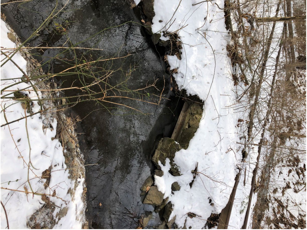
Photo 3. Mortared stone box culvert (#4) near Station 167 + 20 to be replaced
