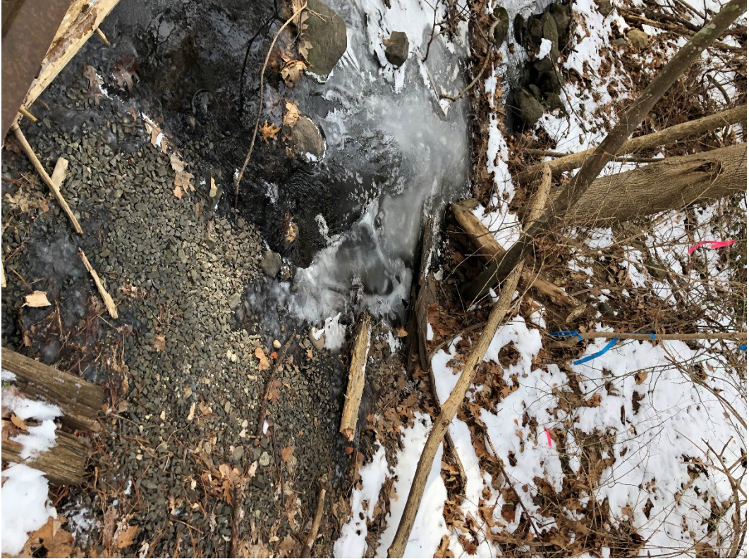
Photo 7. Bank below the railroad track at crossing; stream has cut around the collapsed culvert
