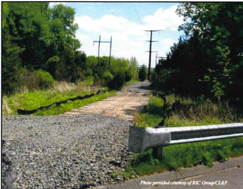
Construction entrance track pad.
