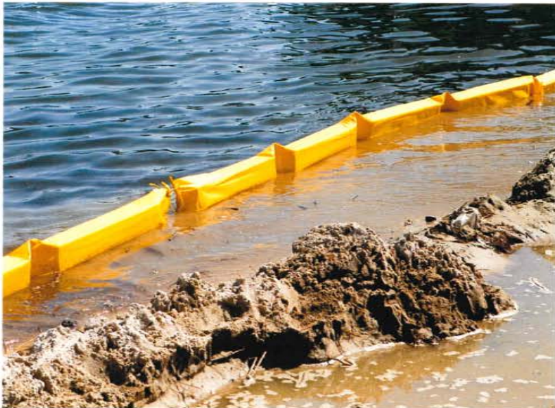
TURBIDITY CURTAIN DETAIL - EROSION CONTROL BARRIER TYPE C (OPTION 2)
