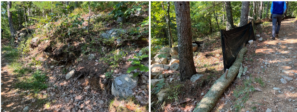
Section of Gen John Nixon Trail to be stabilized. Photo taken 9/9/22.
