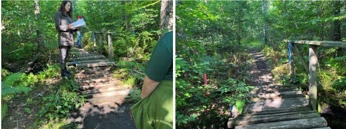
Little Sachem Brook Bridge to be replaced. Photo taken 9/9/22.
