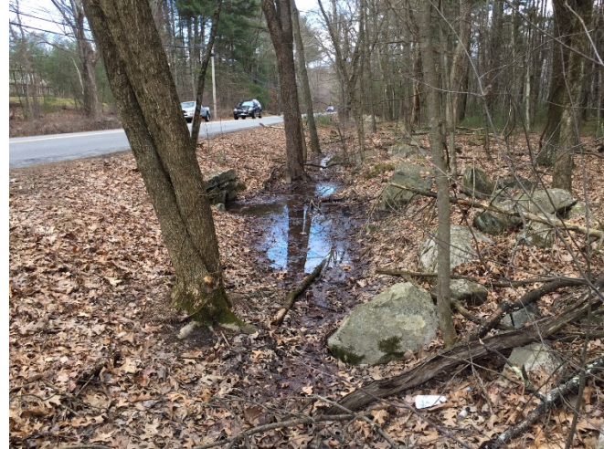
Drain ditch with puddle after rainstorm looking east. (4/1/2022)
