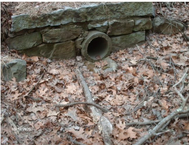
Road drain inlet to ditch. (3/12/2020)
