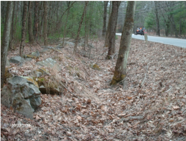
Roadside Drain Ditch (3/12/2020)
