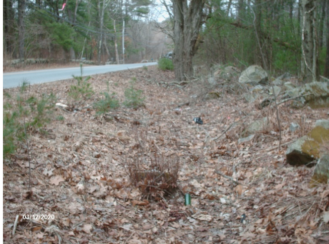
Roadside Drain Ditch (3/12/2020)
