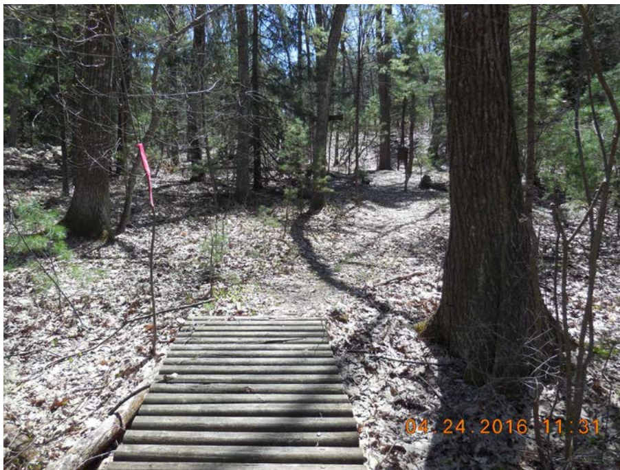
Photograph 36: View of typical footpath boardwalk spanning an intermittent stream
