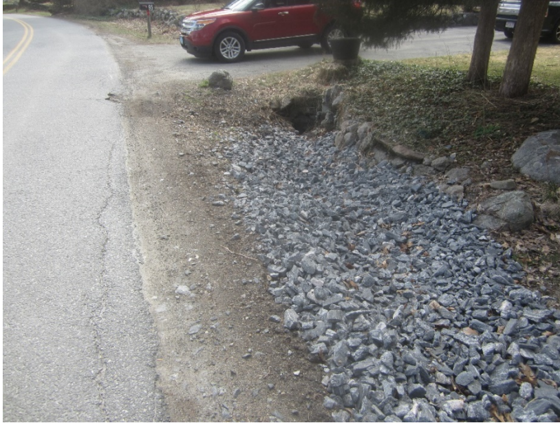
Picture 1 of 2: Roadside channel leading to culvert.
