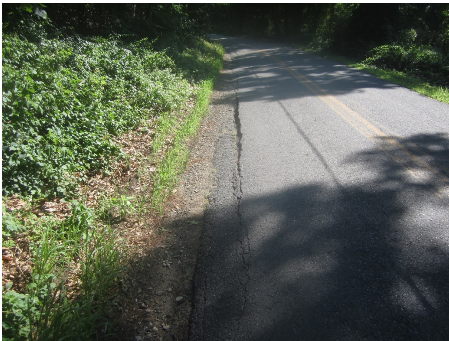
Picture 2: The travel lane measured 7-foot travel where the pavement drops off. We will “carry the line” of the existing pavement on either side of the broken edge of pavement to widen the roadway to its original width.
