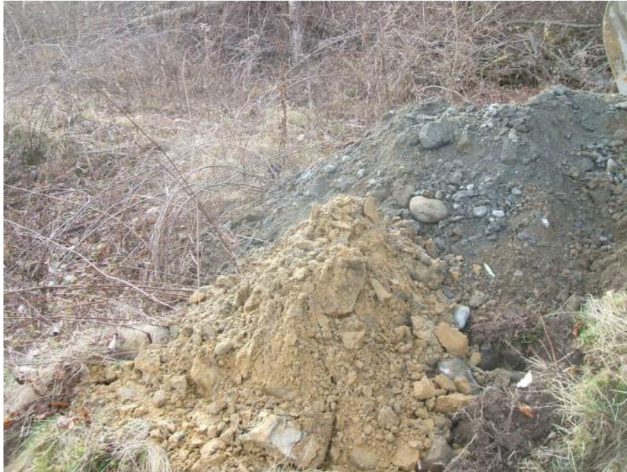
Photo 10: Excavated materials generated from TP-3
