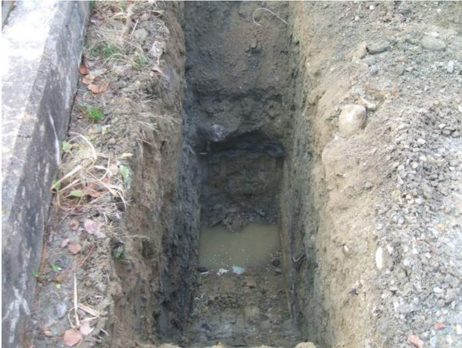
Photo 4: Excavation of TP-2
