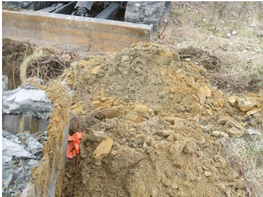
Photo 11: Excavated materials generated from TP-3
