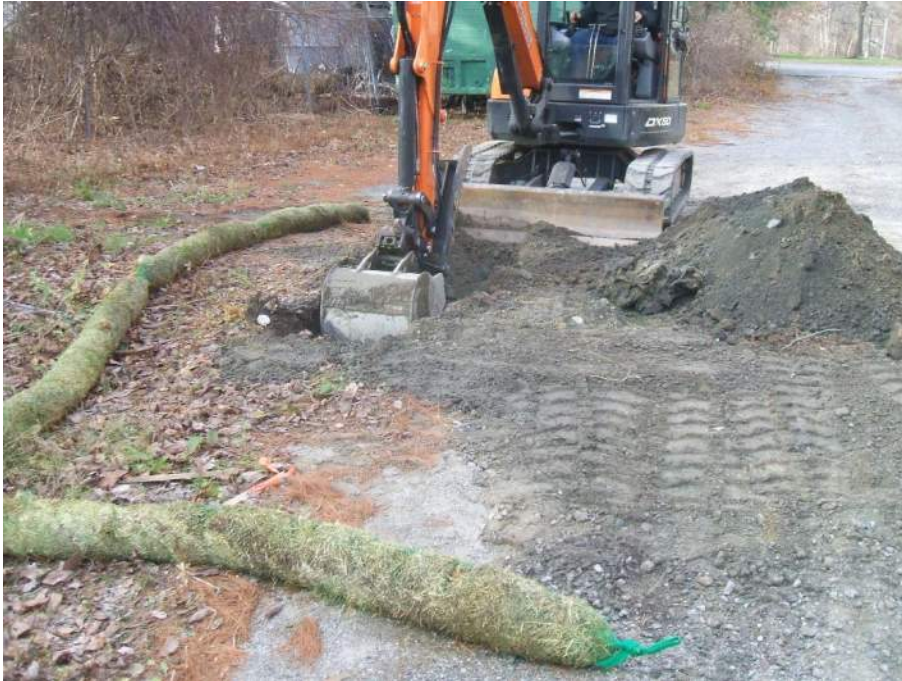
Photo 1: Excavation at TP-1
