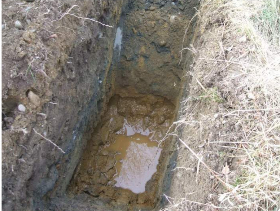
Photo 8: Excavation of TP-3
