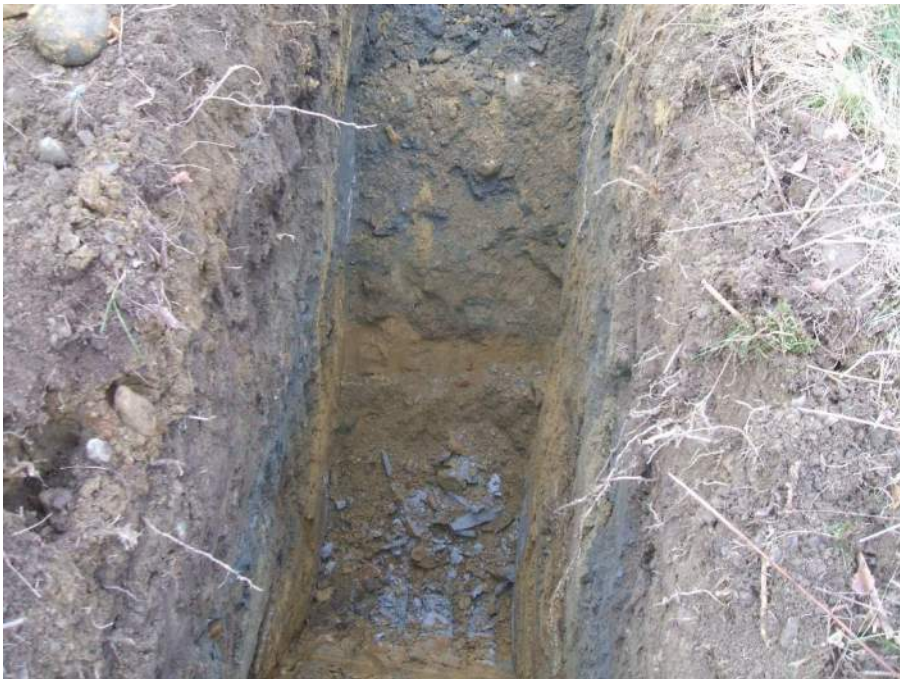
Photo 7: Excavation of TP-3
