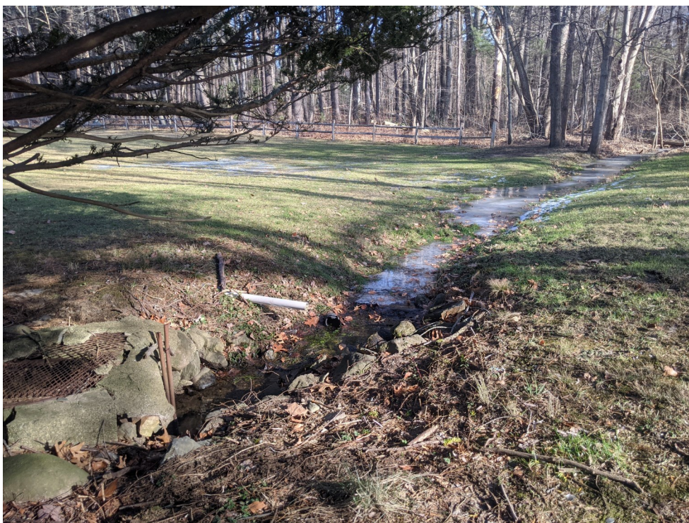
View of the stream downgradient of a forested Bordering Vegetated Wetland; this stream flows into a sub-surface structure and discharges to the 12-inch RCP depicted in Photo 3 - facing east.
