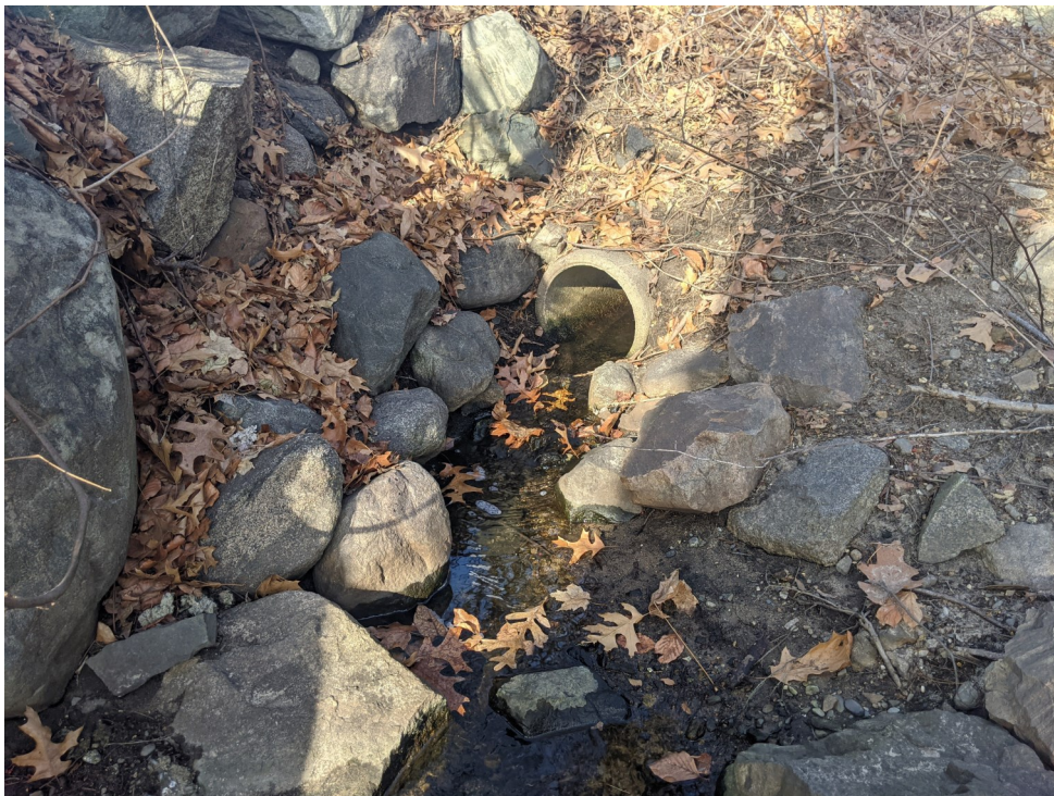
View of the 12-inch RCP that discharges into the B1/B2 Series intermittent stream—facing north.
