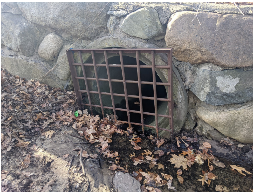
View of the RCP that discharges the stream to the stormwater system under Concord Road—facing west.
