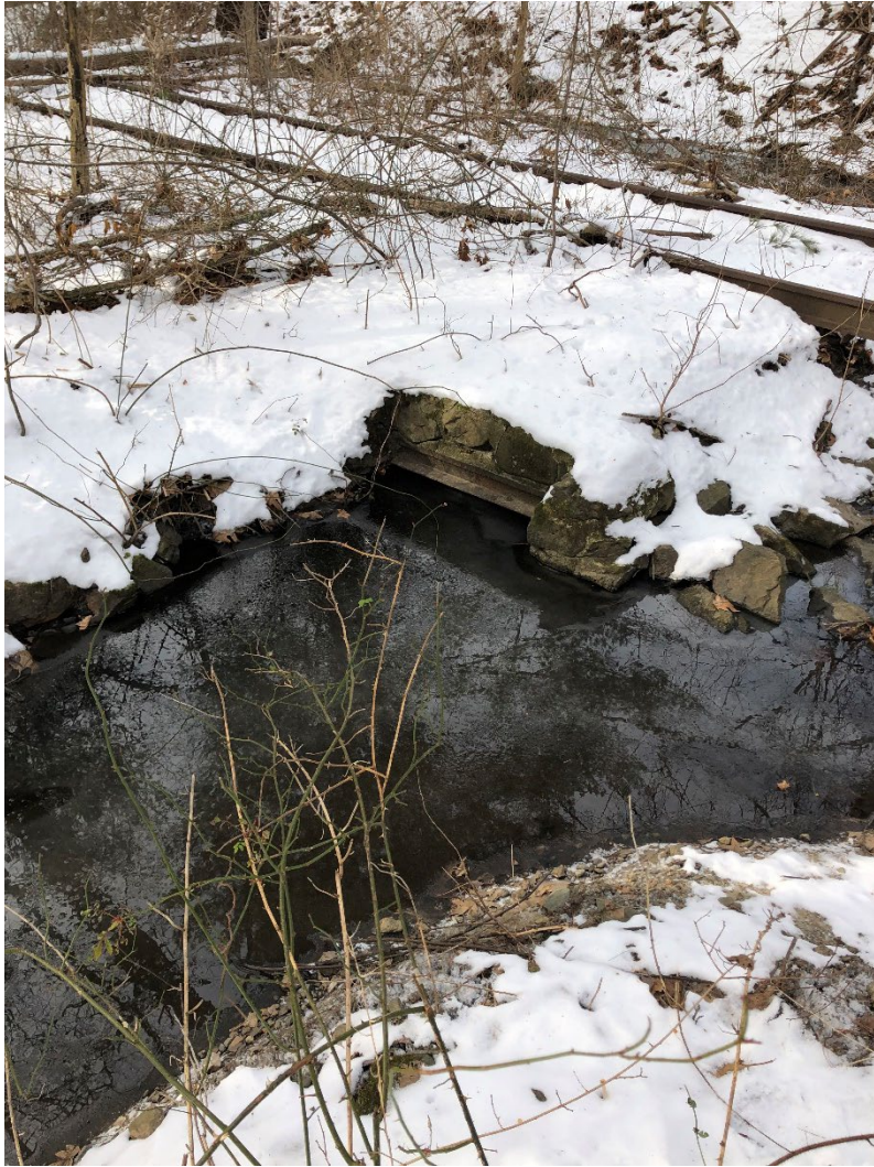
Photo 3. Mortared stone box culvert (#4) near Station 167 + 20 to be replaced
