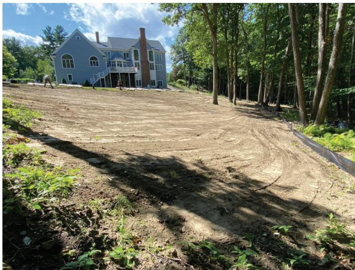
2. After installation of sediment control, we mechanically mowed area and seeded with New England Conservation and Wildlife Seed Mix
