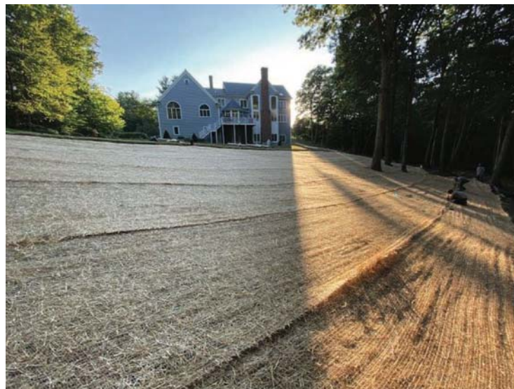
3. Covered exposed loam with straw erosion control blanket: BioNet S75BN and staple into existing slope
