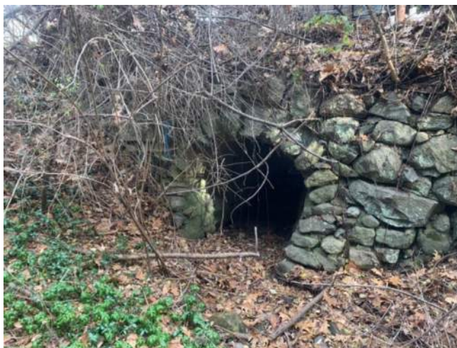
Photograph 1 – stacked stone headwall inlet
