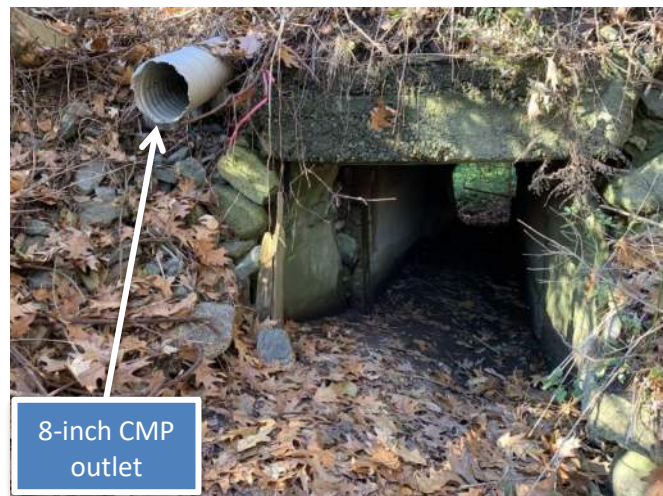
Photograph 2 – concrete and stone outlet opening
