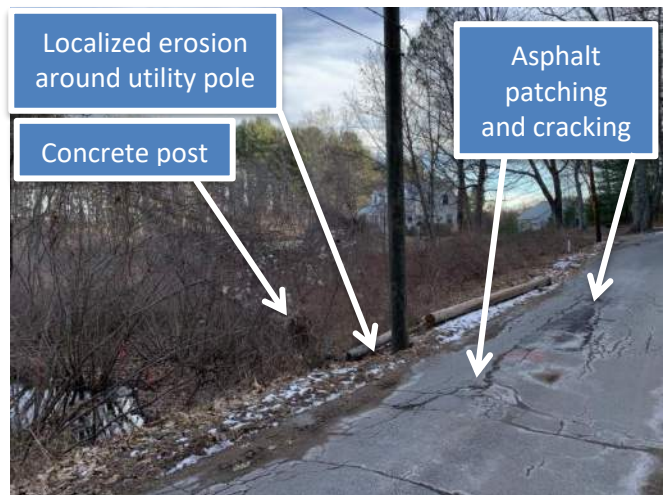
Photograph 4 – localized erosion and cracking
