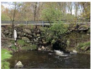
Photo 1 – Retaining stone wall, RCP outlet and CMP
