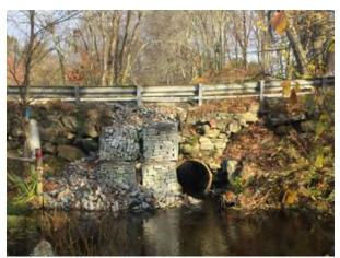
Photo 4 – Installed gabion baskets and rip rap
