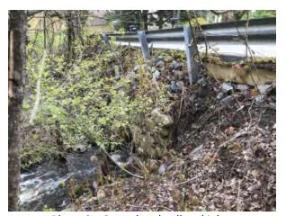
Photo 2 – Stone headwall and inlet
