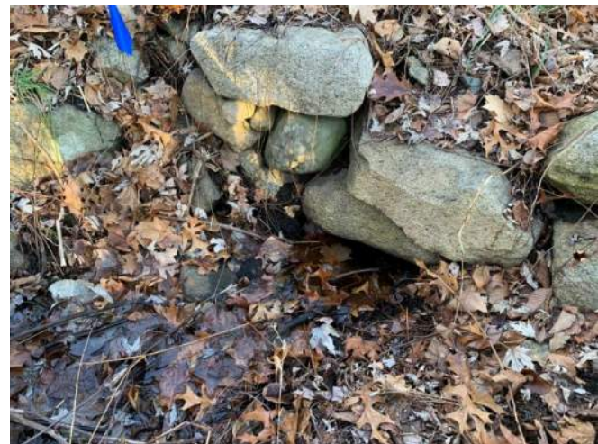
Photograph 2 – Stone headwall Culvert #110 outlet
