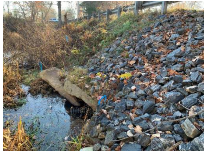
Photograph 4 – Stacked stone headwall Culvert #149 outlet
