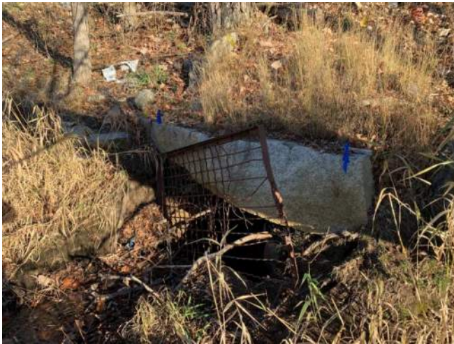
Photograph 3 – Stone headwall Culvert # 149 inlet
