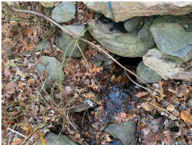
Photograph 1 – Stone headwall Culvert # 110 inlet
