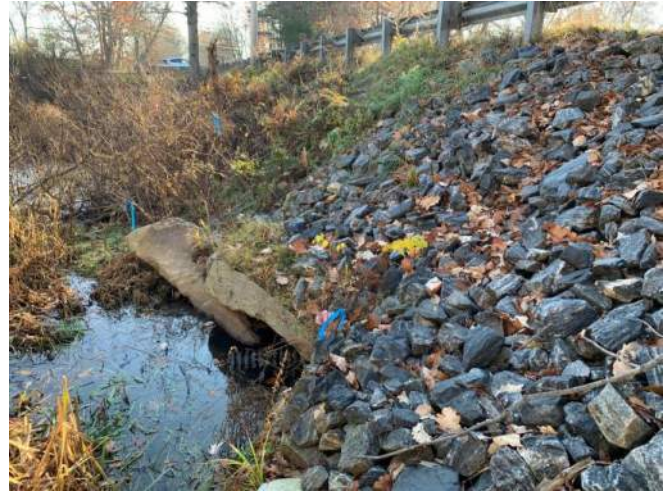
Photograph 4 – Stacked stone headwall Culvert #149 outlet
