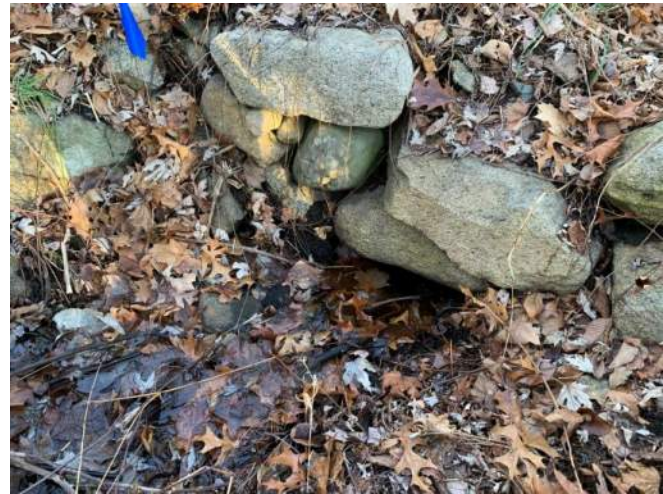
Photograph 2 – Stone headwall Culvert #110 outlet
