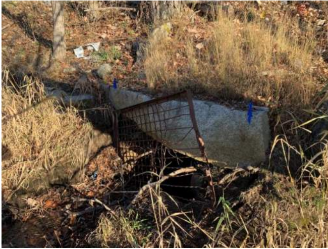
Photograph 3 – Stone headwall Culvert # 149 inlet
