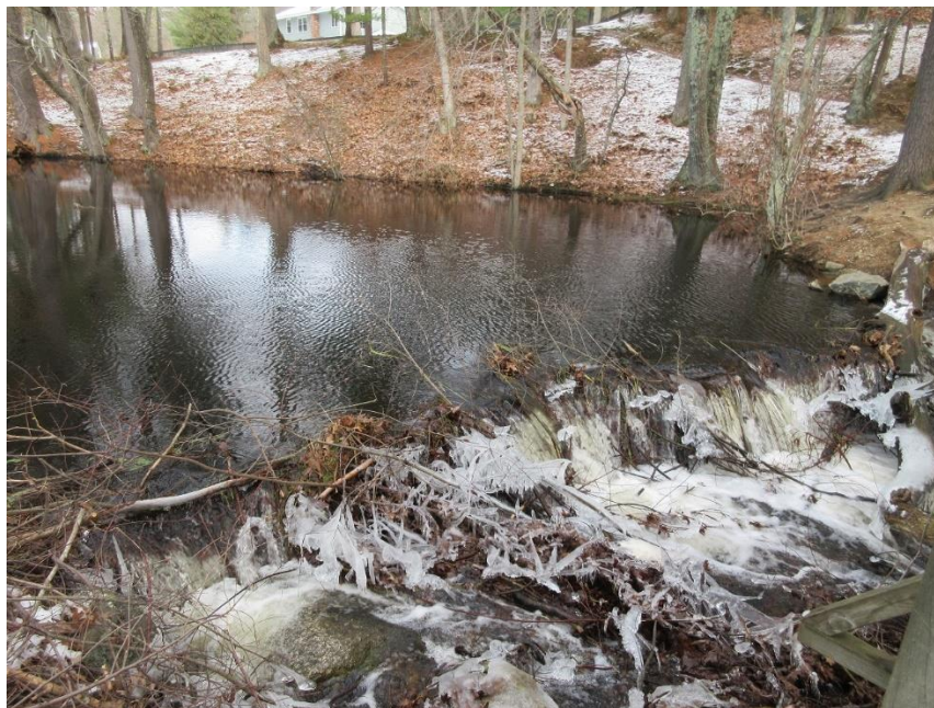
Dam along Hop Brook
