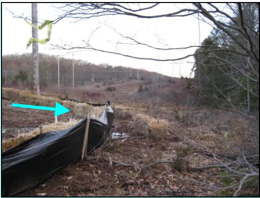
Properly installed hay bale barrier with silt fence.
