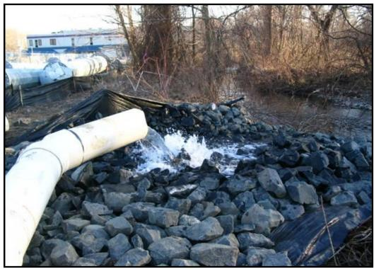
Riprap underlain by geotextile fabric
