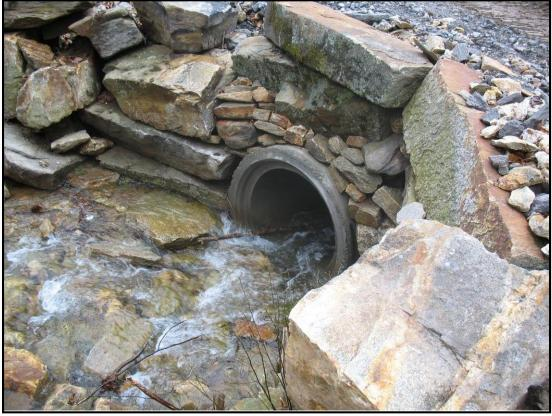
Culvert and riprap for stream crossing.
