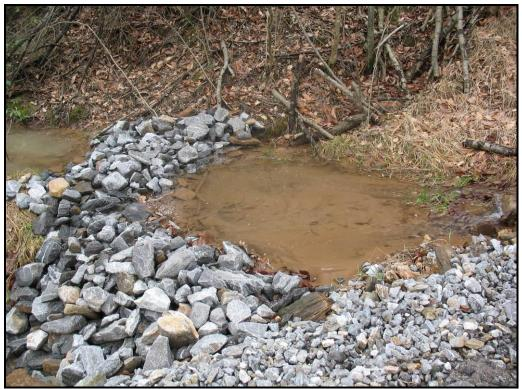
Stone check dam at construction site.
