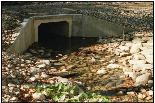
Embedded box culvert with wing walls.
