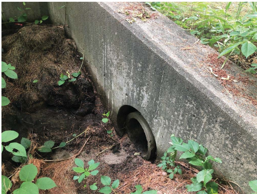
Photo 2: Stormwater inlet to stormwater detention basin
