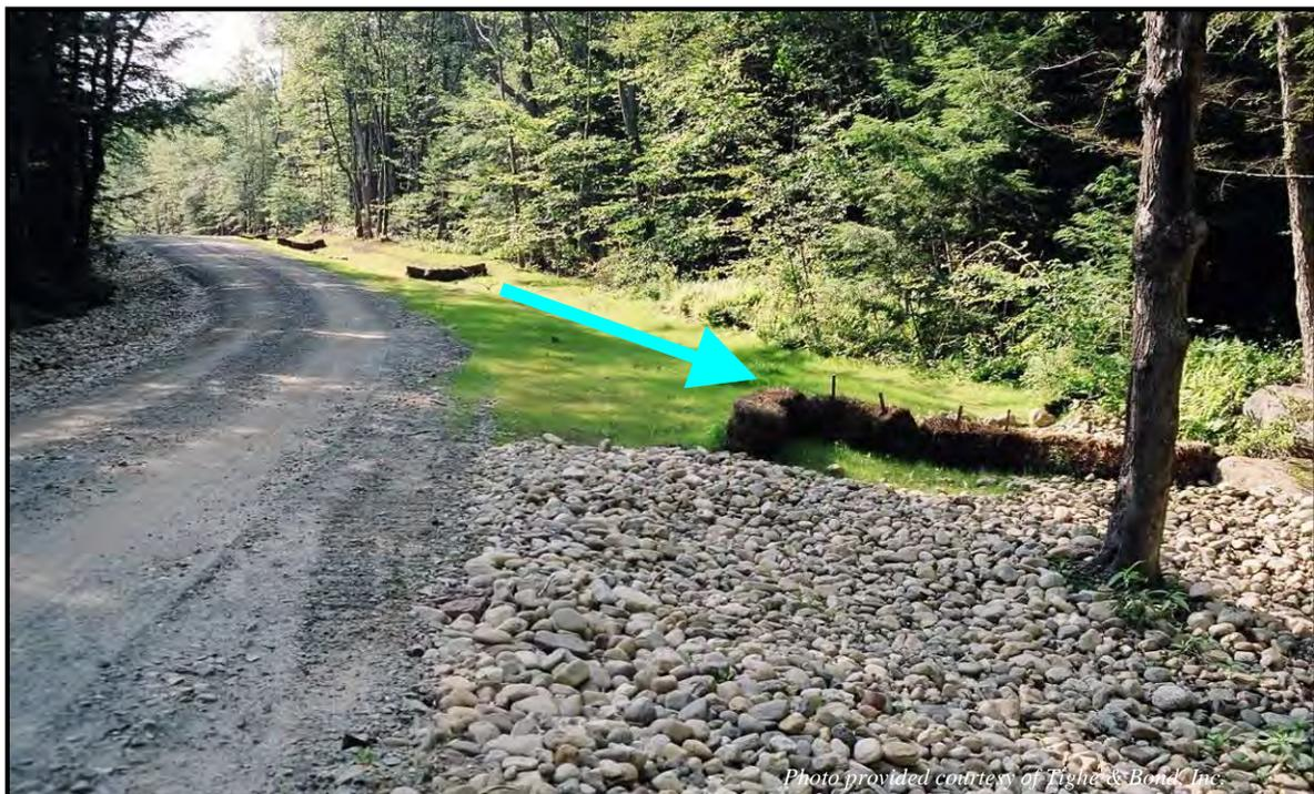
Grass-lined swale underlain with erosion control blanket and containing hay bale check dams; used to quickly stabilize soils along a construction access road subjected to significant stormwater runoff. Blue arrow indicates direction of flow.
