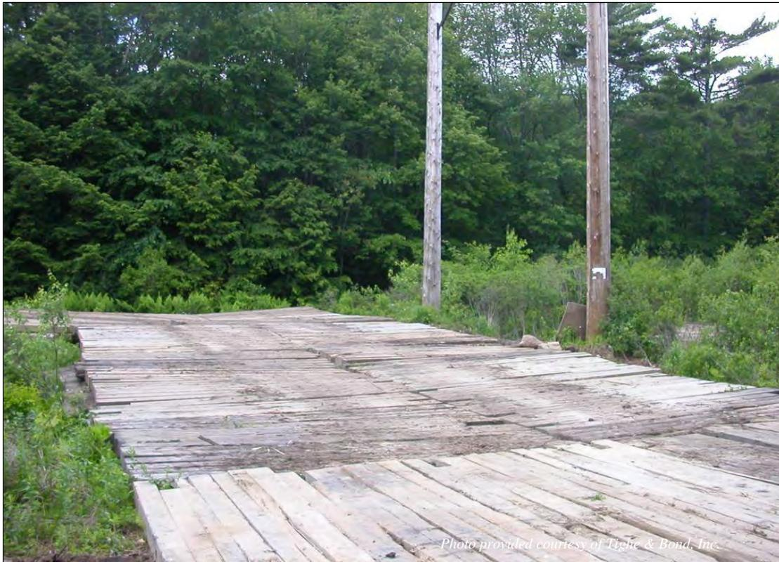
Construction mat wetland work-pad for de-energized work.
