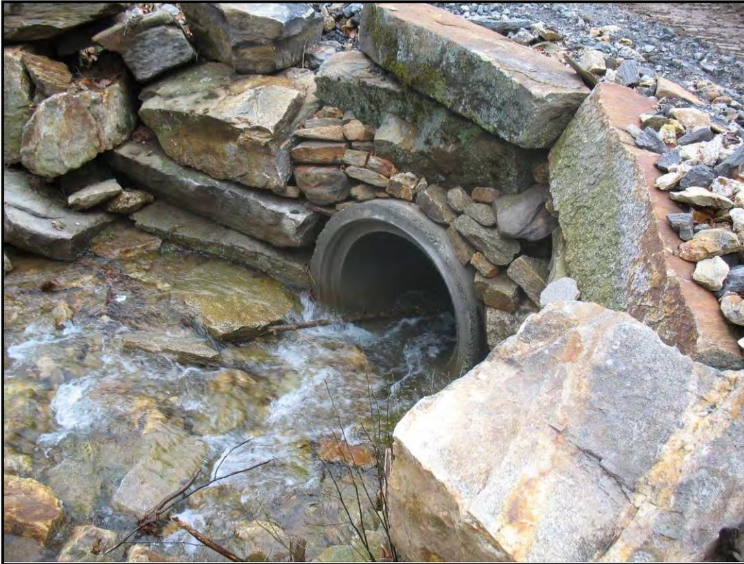
Culvert and riprap for stream crossing.
