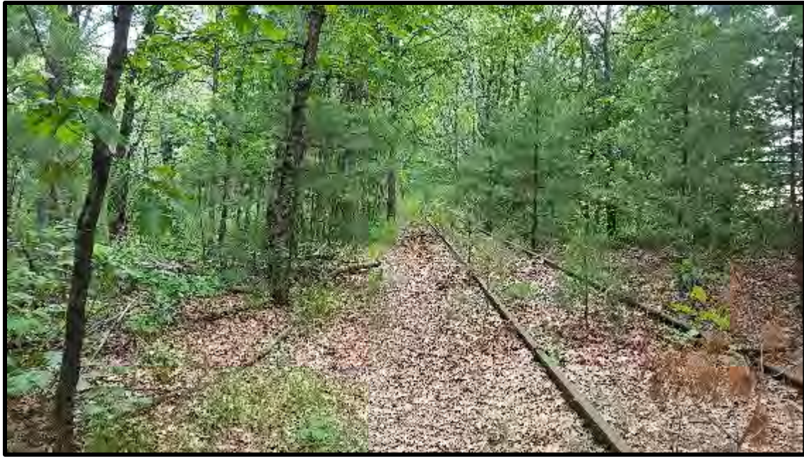
Photo 7 Looking east down the ROW near Station 576+30 with a moderately defined foot path visible in the right side of the photograph. This location is between Horse Pond Road and Union Avenue.
