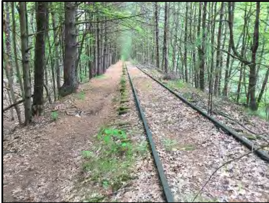
Photo 5 Looking east down the ROW near Station 535+50 with the well-defined foot path visible in the left side of the photograph. This location is between Peakham Road and Horse Pond Road.
