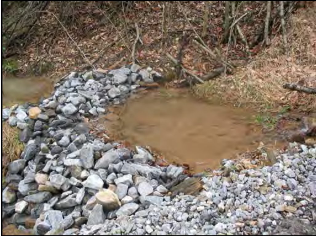
Stone check dam at construction site.
