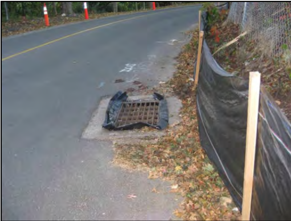
Catchbasin protected from sedimentation by filter fabric.
