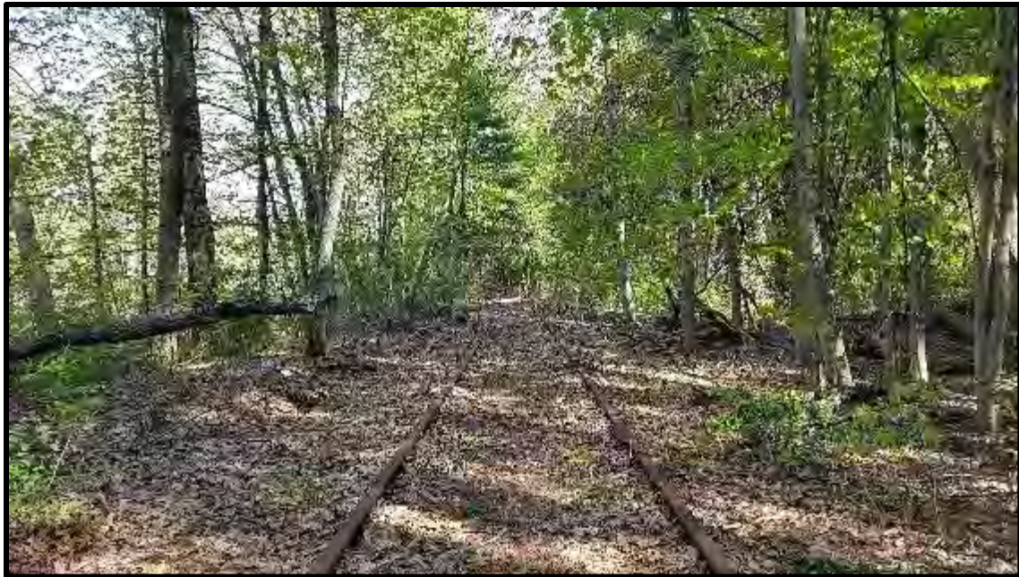
Photo 8 Looking east down the ROW near Station 717+90. This location is between Boston Post Road and Hop Brook.
