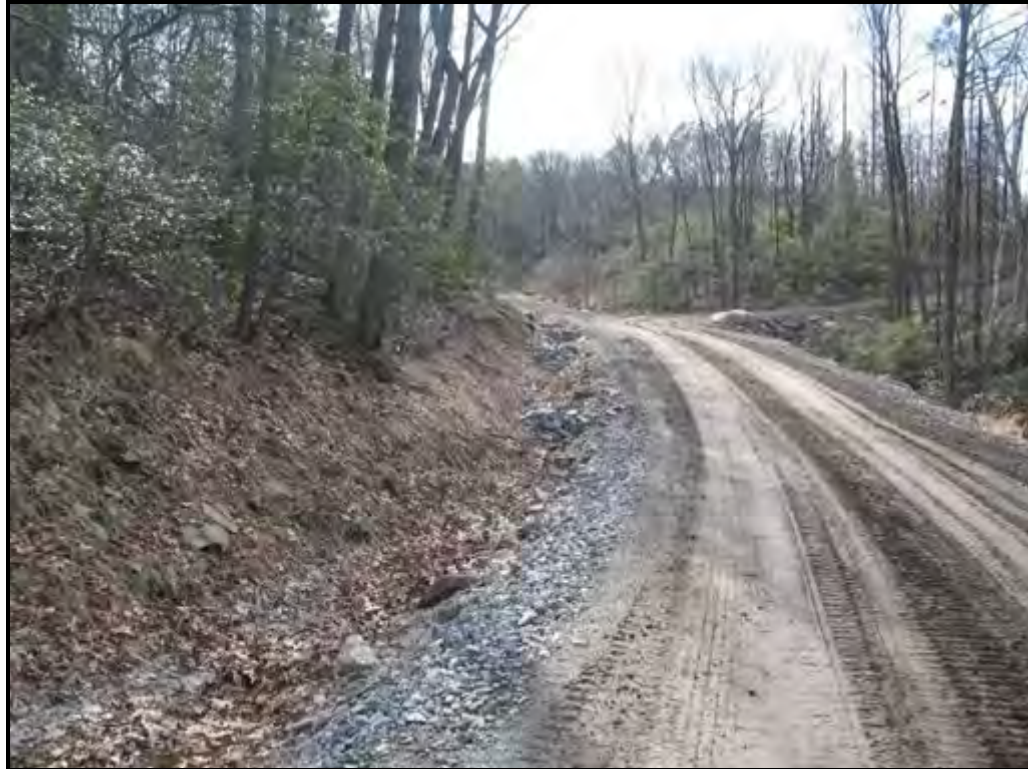
Stone check dams at construction site.
