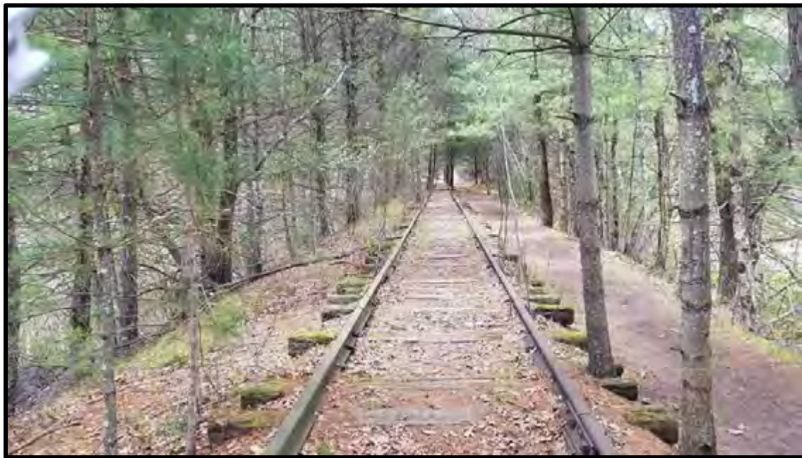
Photo 2 Looking west down the ROW near Station 399+00 with the well-defined foot path visible in the right side of the photograph. This location is west of Dutton Road and Hop Brook.
