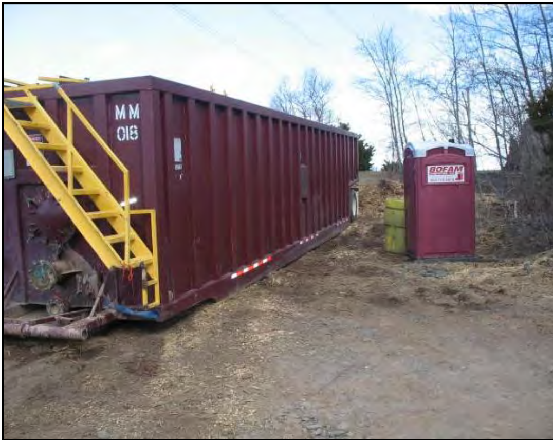
Frac tank on-site for dewatering activities.
