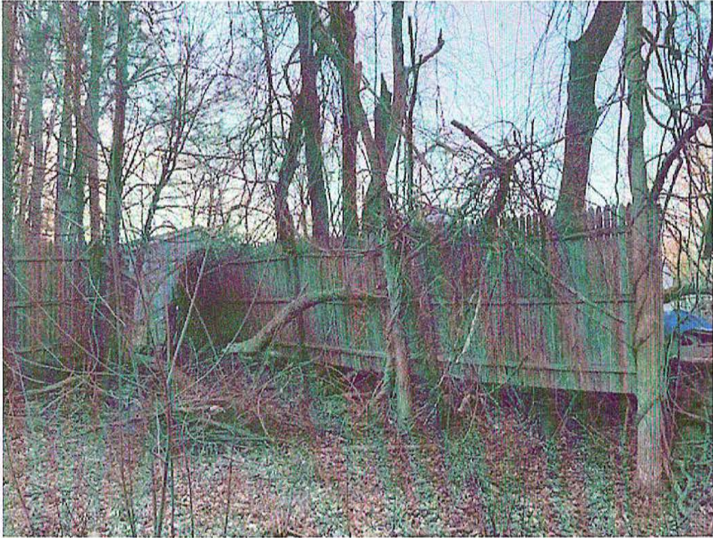
Fence view #2 showing Bittersweet damage
