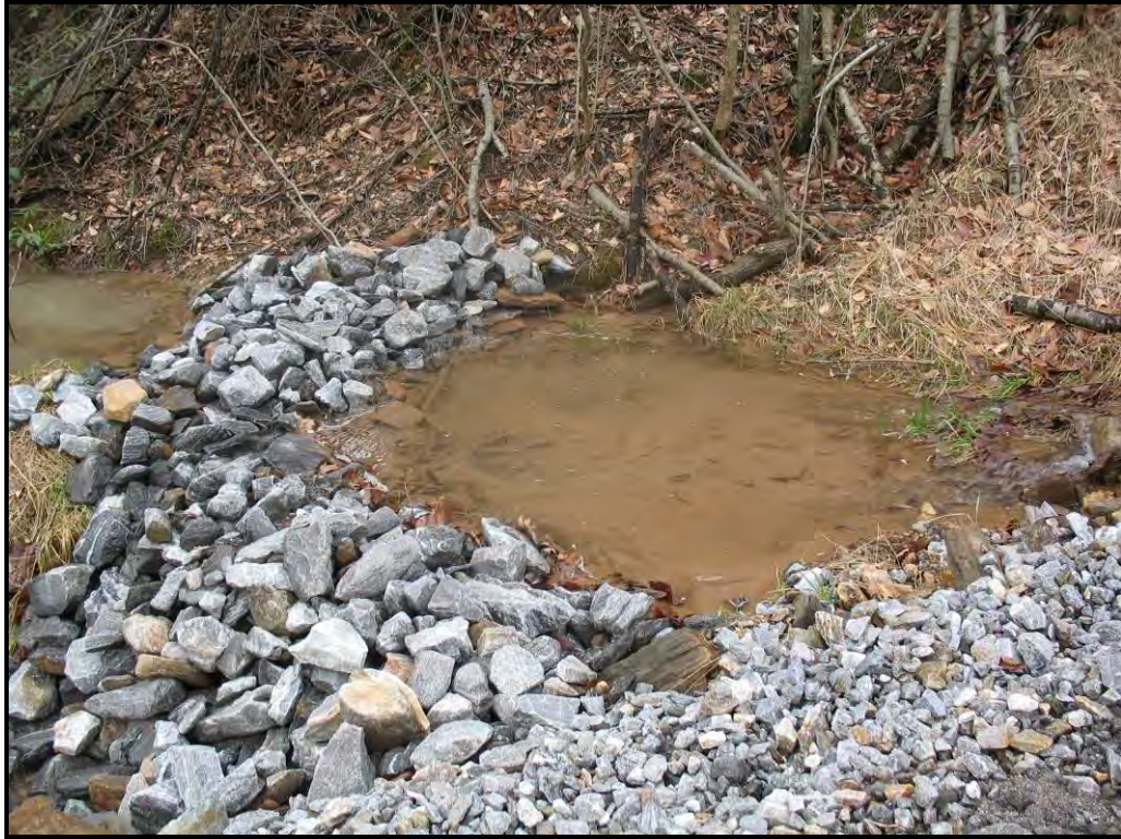
Stone check dam at construction site.
