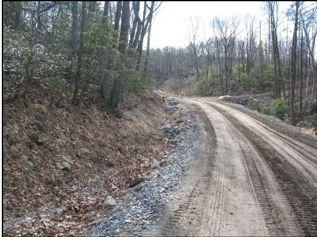
Stone check dams at construction site.
