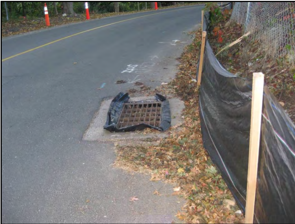
Catchbasin protected from sedimentation by filter fabric.
