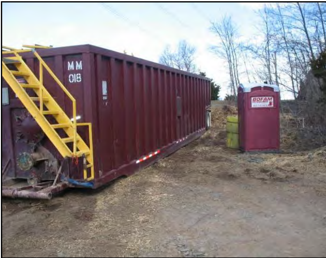
Frac tank on-site for dewatering activities.
