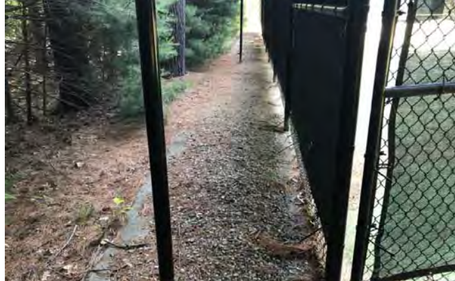
Photo of the 3-foot gravel apron adjacent to the turf tennis court that provides stormwater infiltration
