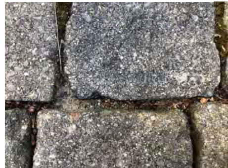
Photo of the sand filled patio joints
