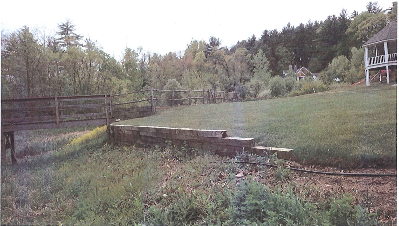
Photo 2 - PISMP area north of existing bridge.
