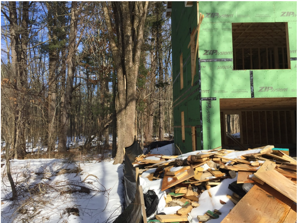
Photo 3 - Base of Tree #1, located outside of erosion control barrier.
