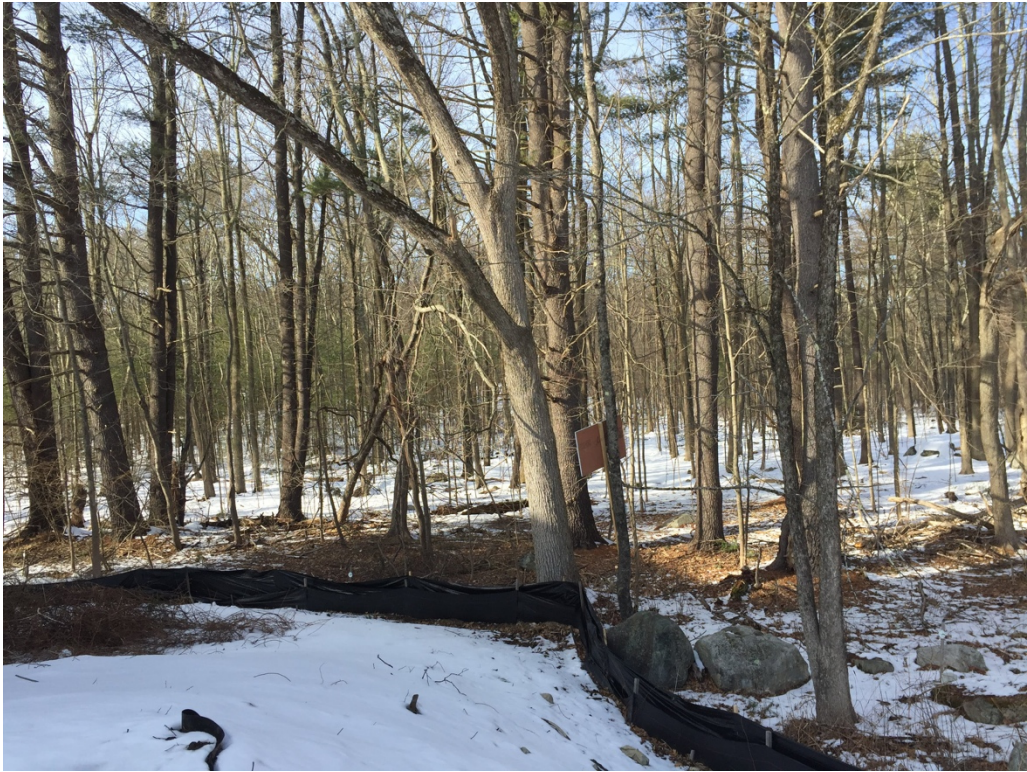
Photo 5 - Base of Tree #2, located outside of erosion control barrier and view of lower (overhanging) branch.
