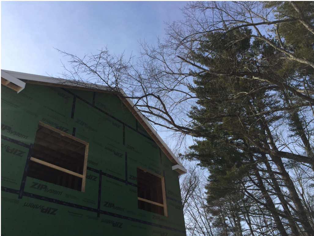
Photo 4 - Overhanging branch to be removed from Tree #2, located northeast of house.
