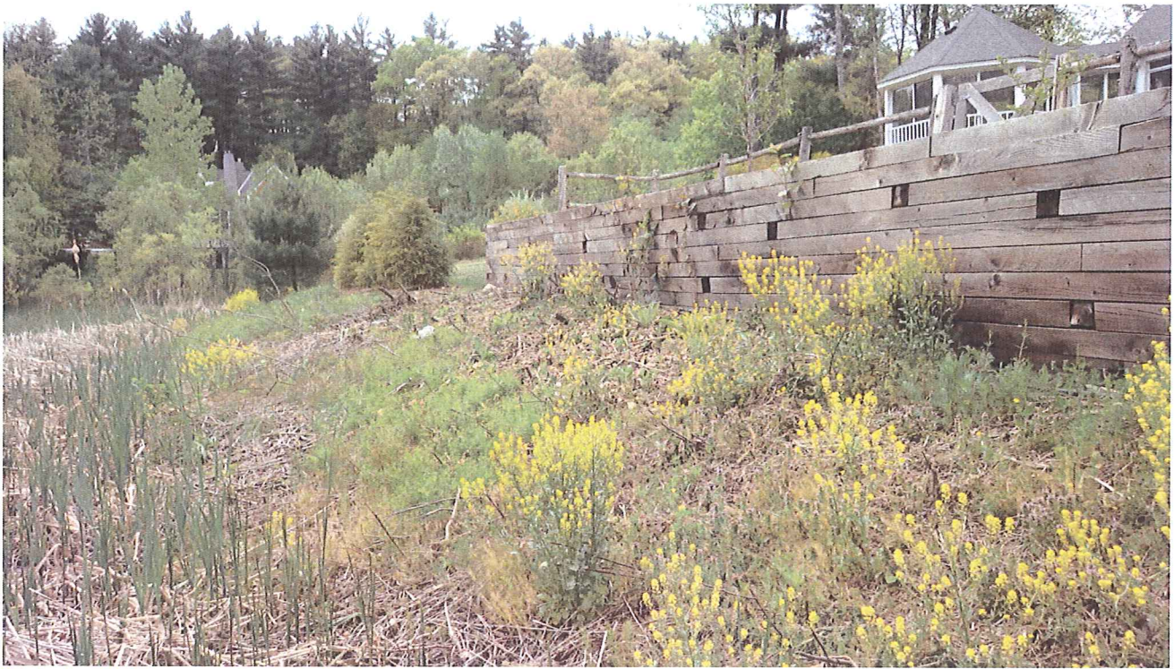
Photo 1 - PISMP area west of existing bridge.
