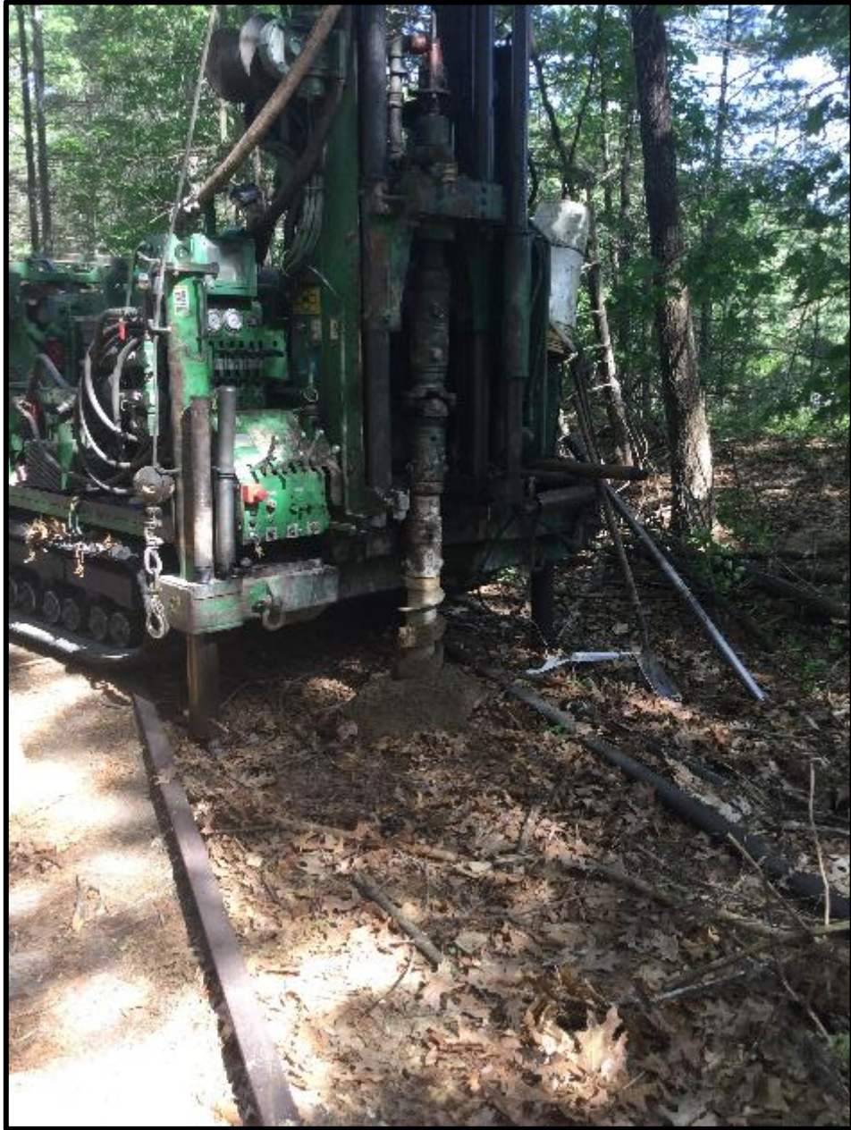
Representative photo of the drill rig advancing a boring
