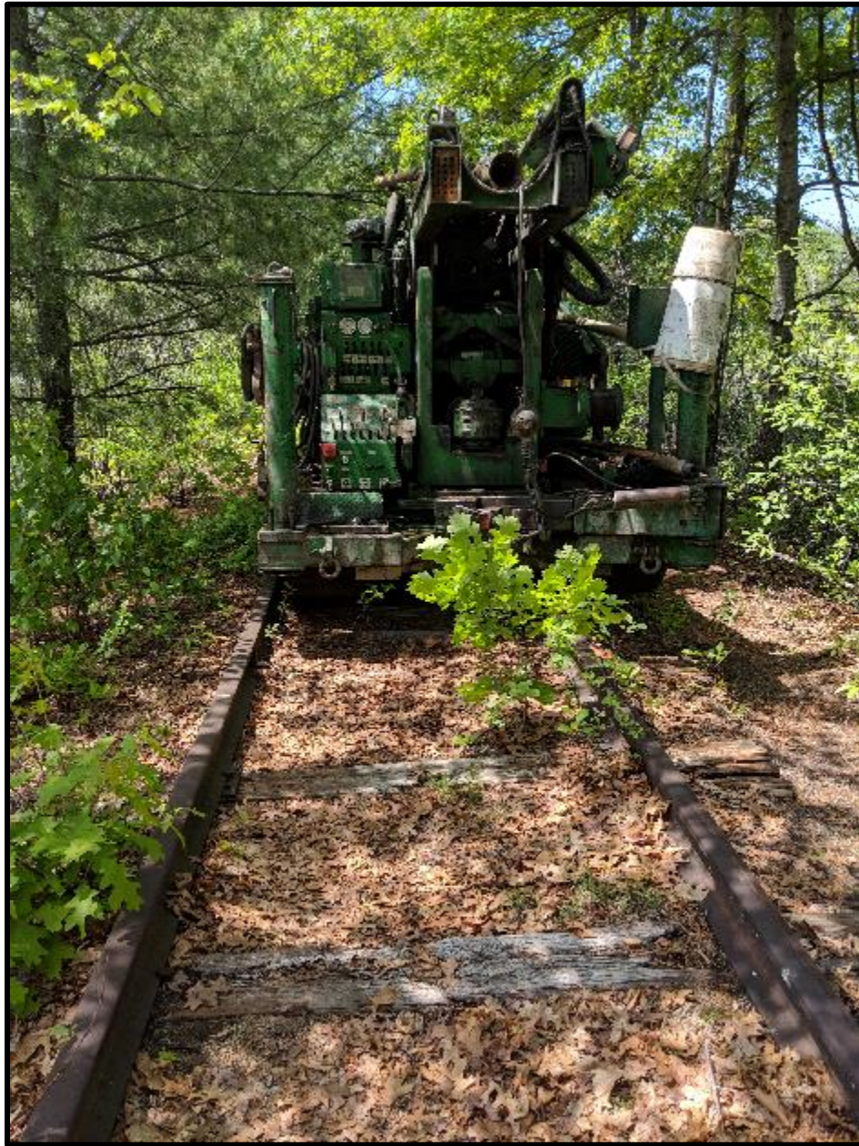
Representative photo of the drill rig maneuvering down the ROW
