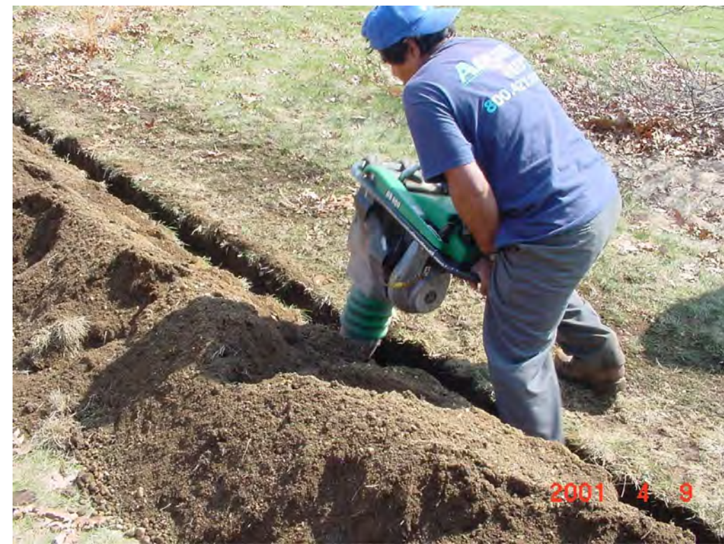
C Installation Example Trench Backfill Compaction
