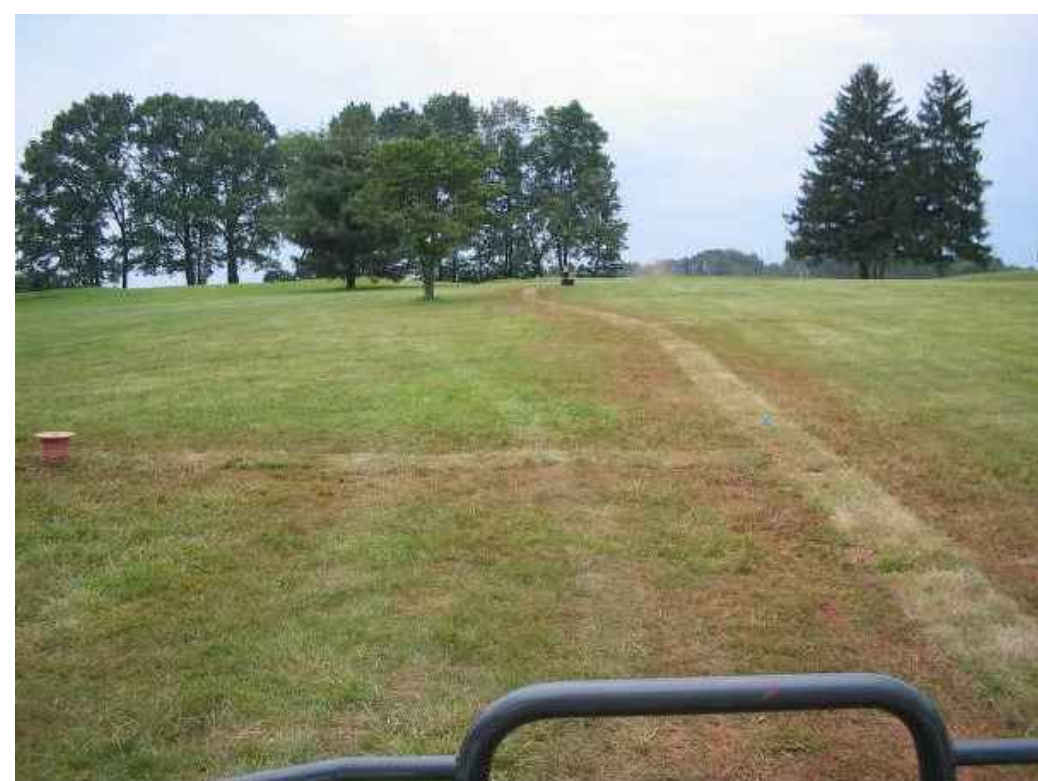
E Installation Example Completed Trench
