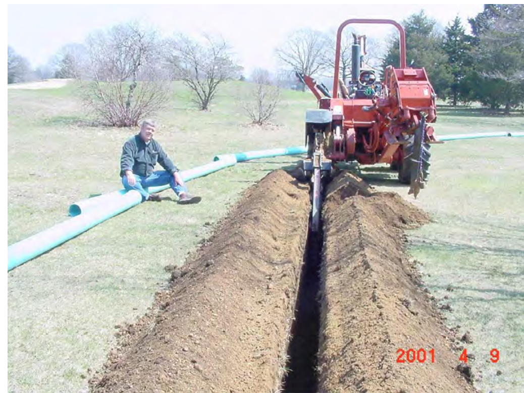
B Installation Example Mainline Trench
