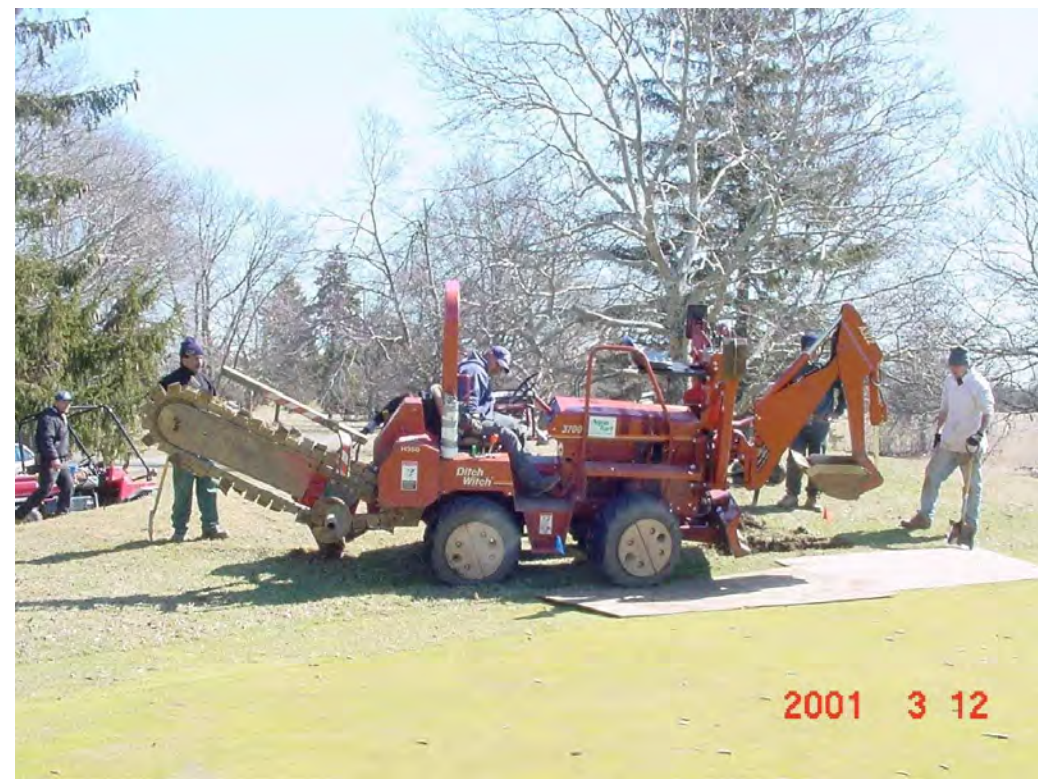
A Installation Example Trenching Machine
