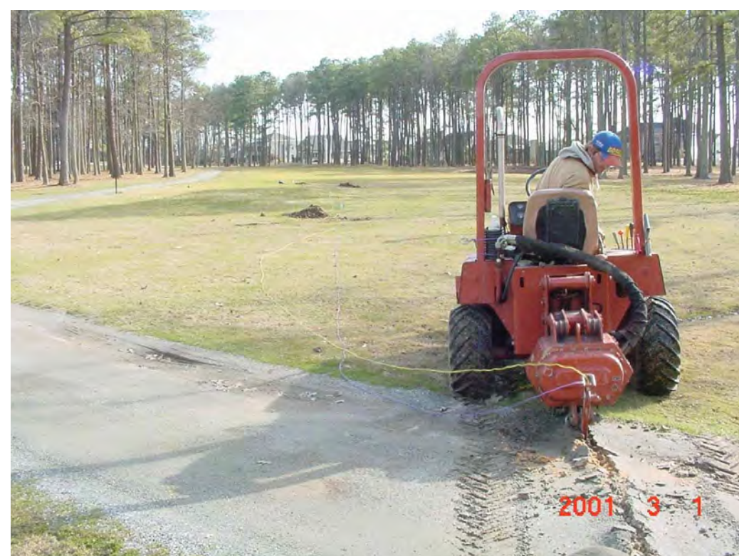
F Installation Example Lateral Pipe Puller
