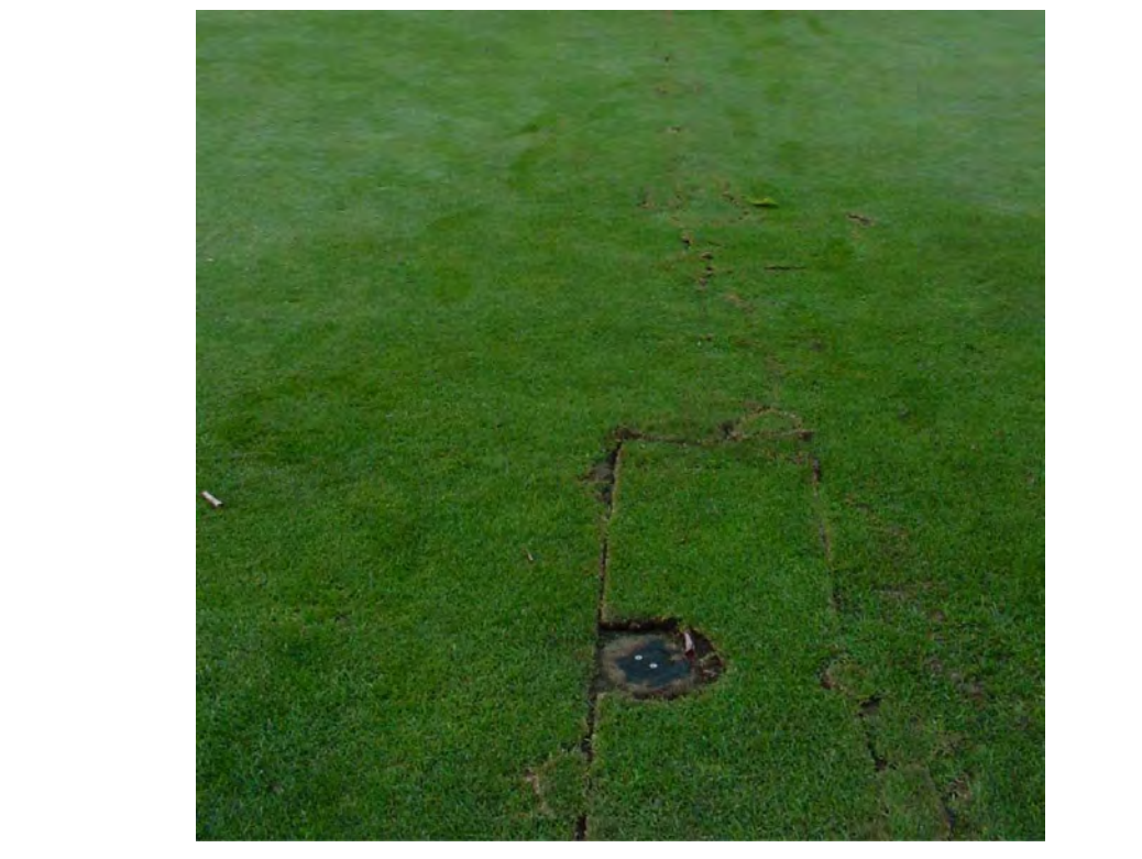
H Installation Example Finished Lateral Pipe Installation
