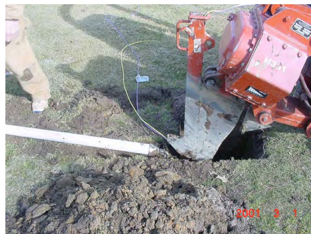
G Installation Example Pulled Lateral Pipe
