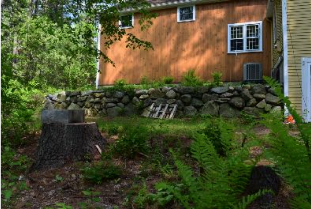
CUT STUMPS IMMEDIATELY ADJACENT TO PATIO AND HOUSE
