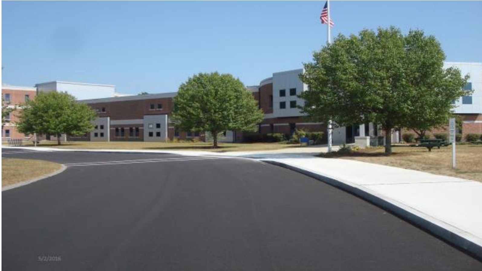
The finished site improvements at Curtis School 2015
