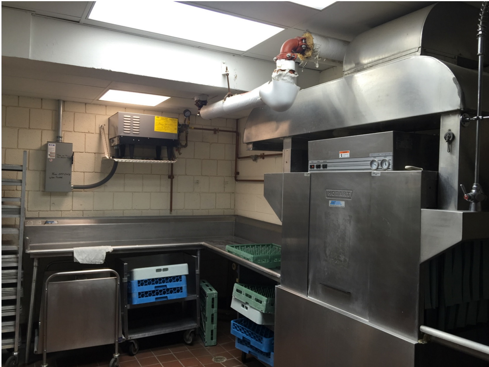
Picture of a dishwasher with hot water booster
