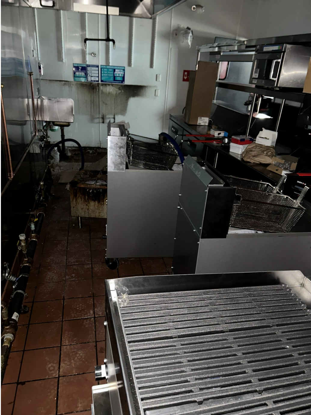
Photo taken by Building Department during inspection on 2/20/2026
