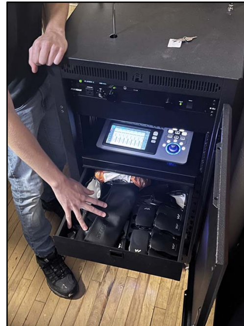
Example of New AV Racks with Assisted Listening Systems Peter Noyes Elementary School
