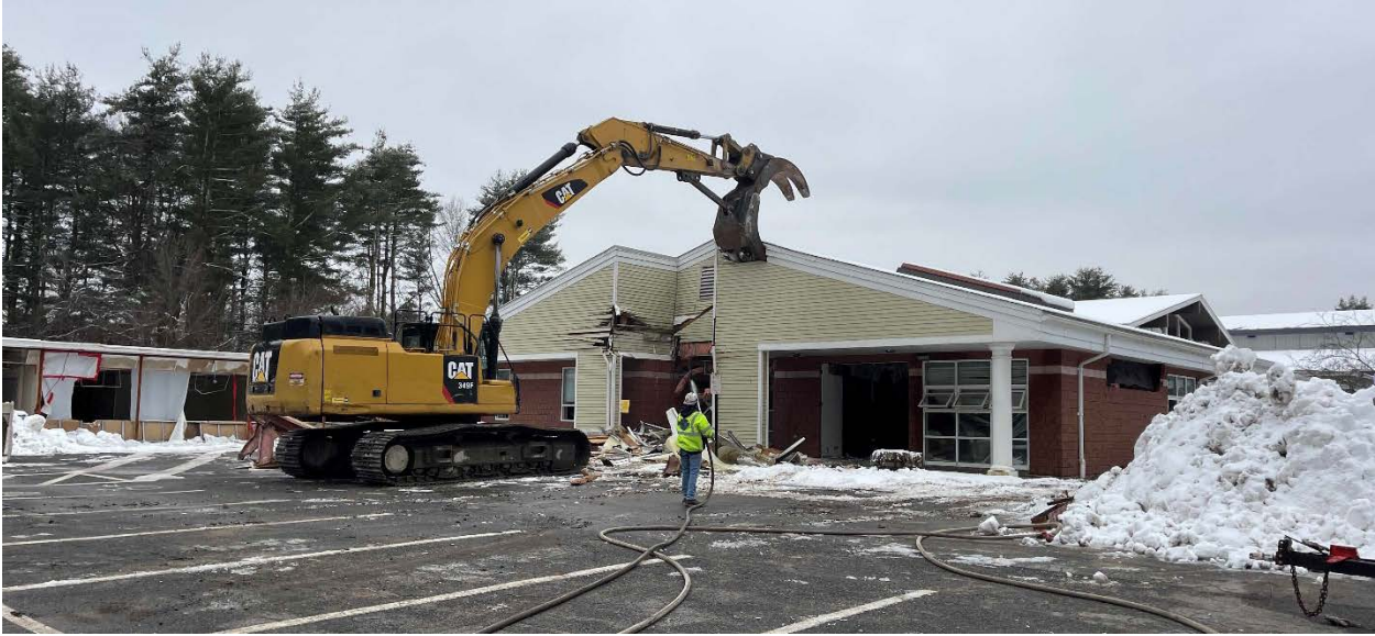
After remediation of asbestos and other materials was completed at the end of January, the school wing was a shell of its former self, and the Senior Center demolition began.
