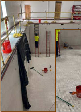
Pool basins Grouting (approx. 7,825 SF)
