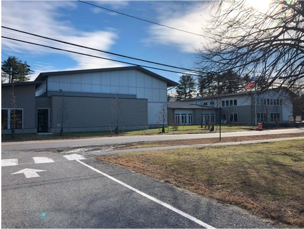
The gym and temporary Park and Rec entry just to its left. The new permanent entrance will be completed as part of the Phase 2 work, after demolition of the old building.
