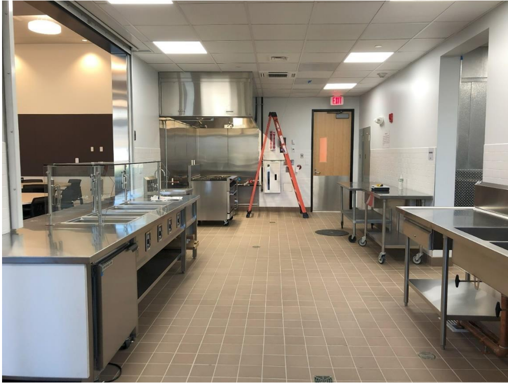
The commercial kitchen with serving counter opening to the Multipurpose room.
