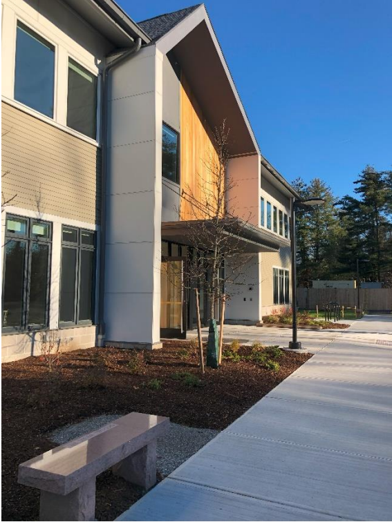
The benches that were outside the Senior Center entrance have been salvaged and reinstalled along the new entrance walk.
