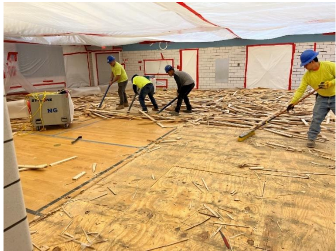
Removing the gym flooring.
