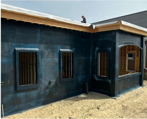
Exterior Sheathing Air-Vapor Barrier, Roofing & HVAC Units
