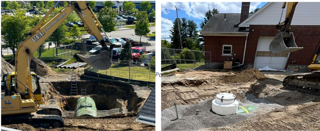
Tight Tank Installation
