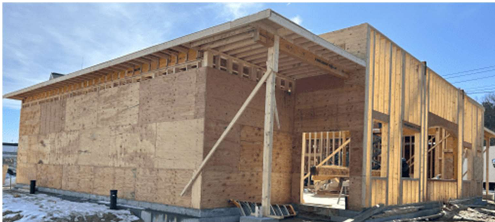
Foundation & Wood Framing
