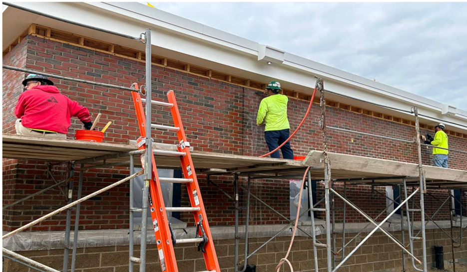
Exterior Siding, Masonry Veneer and PVC Trim
