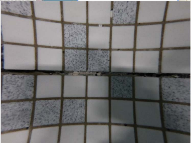
Atkinson Pool Existing Piping & Grout Photos
