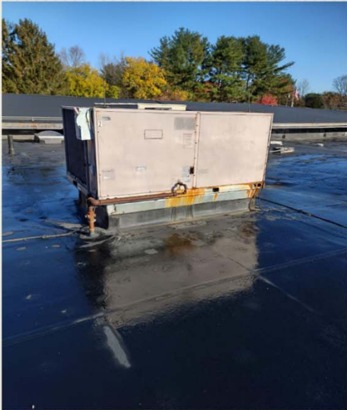
Haynes Media RTU HVAC Replacement
