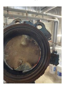
In our recommendation it should be noted that both pools need a fully new grout within the pools and the return penetrations be parged and fittings addressed. The valves within the mechanical room on both the lap and dive pools should all be replaced.
