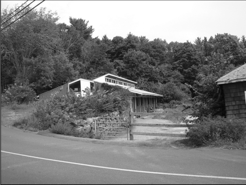
#350 – Barn over Cellar Hole on north side of Morse Road
