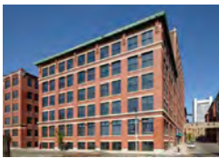
Factory 63: LEED Gold certified
