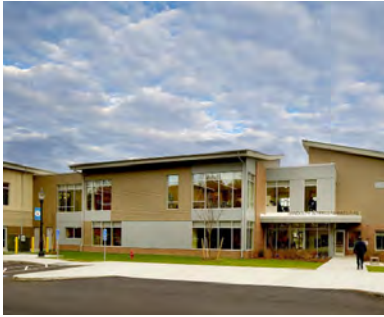
Intergenerational Community Center Randolph, MA
