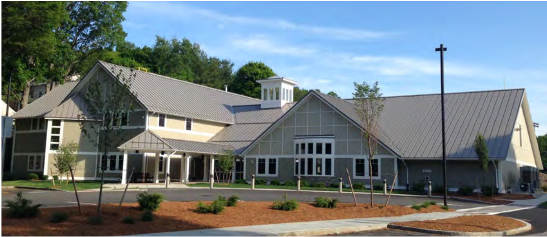
Marlborough Senior Center Marlborough, MA
