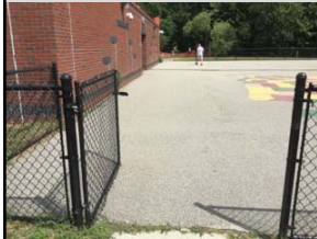
Playground Gate at Nixon School
