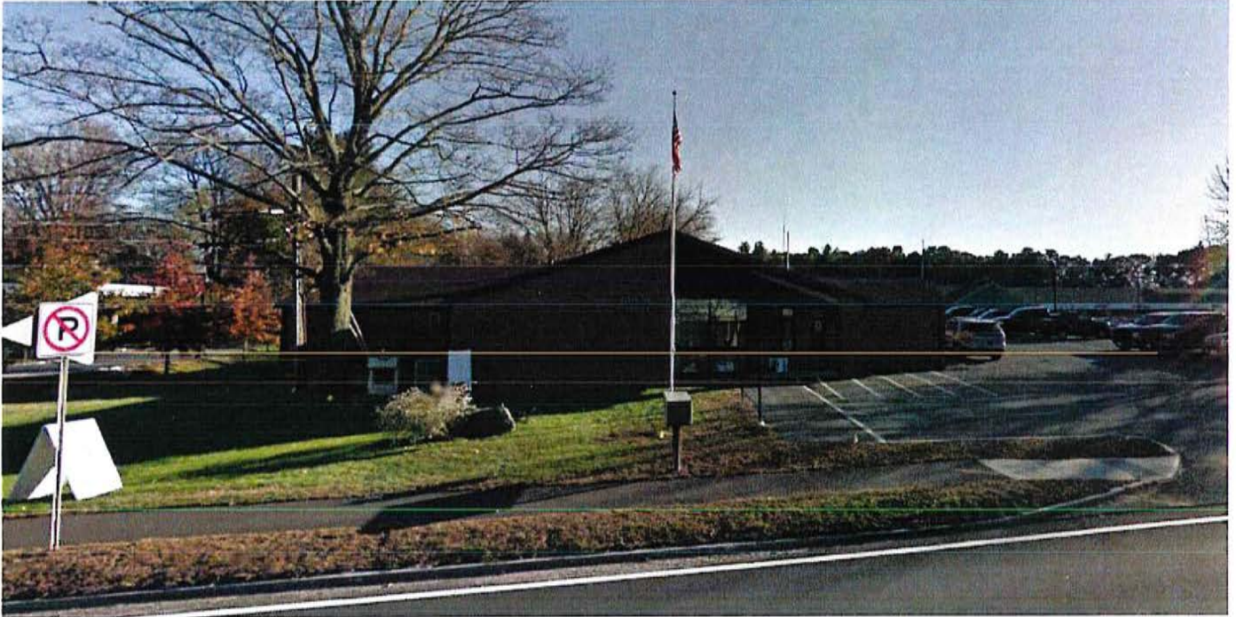
415 Boston Post Road | Front View of Site
