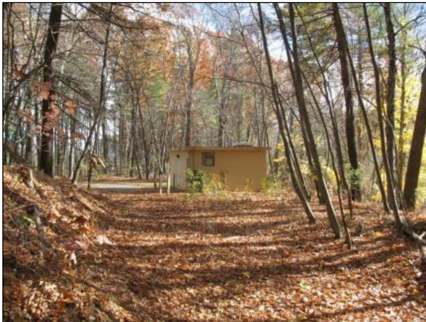
Concord White Pond Well – view south
