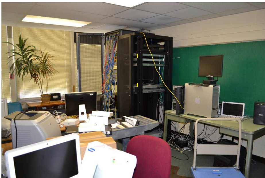
Server and work area
