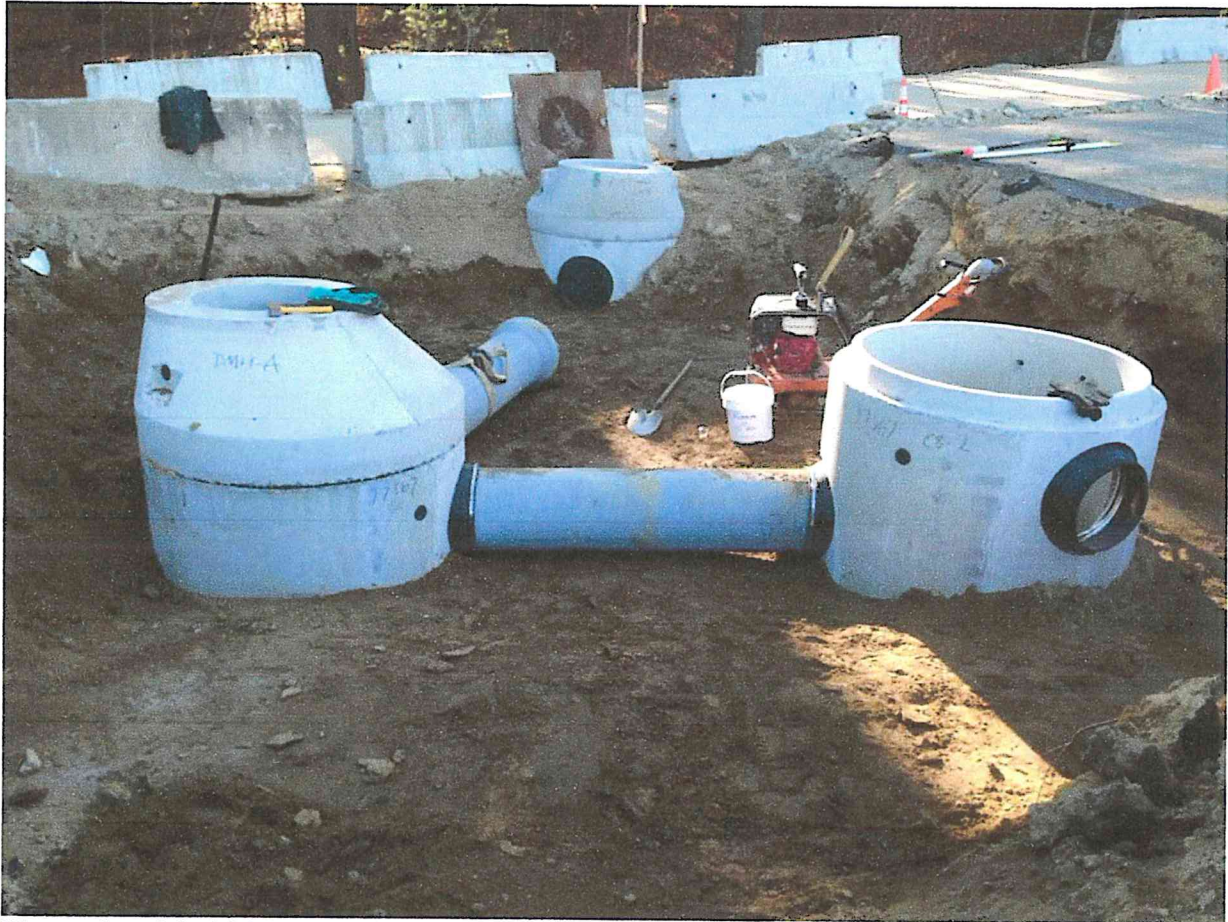
November 20, 2014 – Installation of Drainage Structures (DMH A, CB-1, CB-2) and interconnecting pipe at Musketahquid Drive
