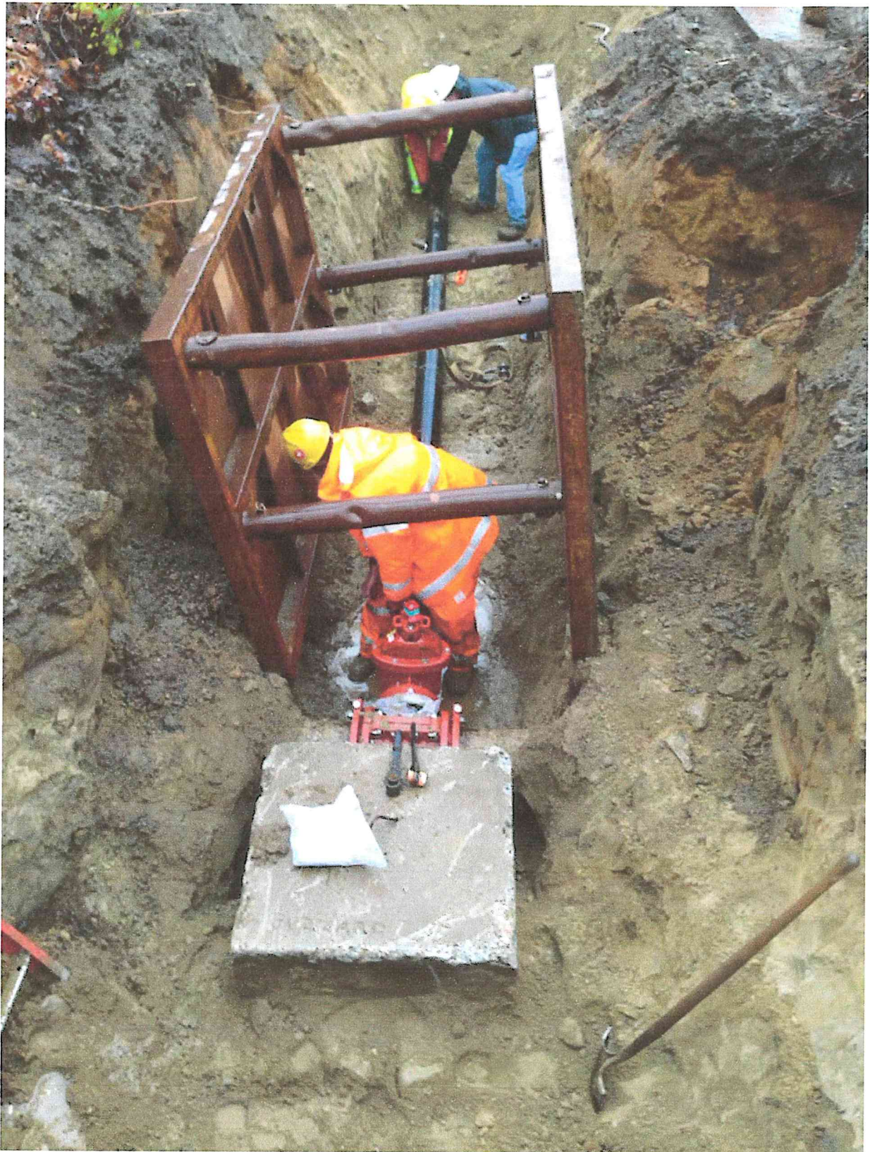
November 17, 2014 – Water Service Connection @ Hudson Road
