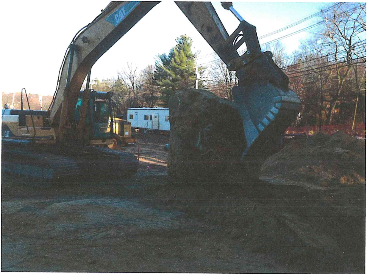
November 14, 2014 – Rock Removal from Musketequid Drive adjacent to Hudson Road
