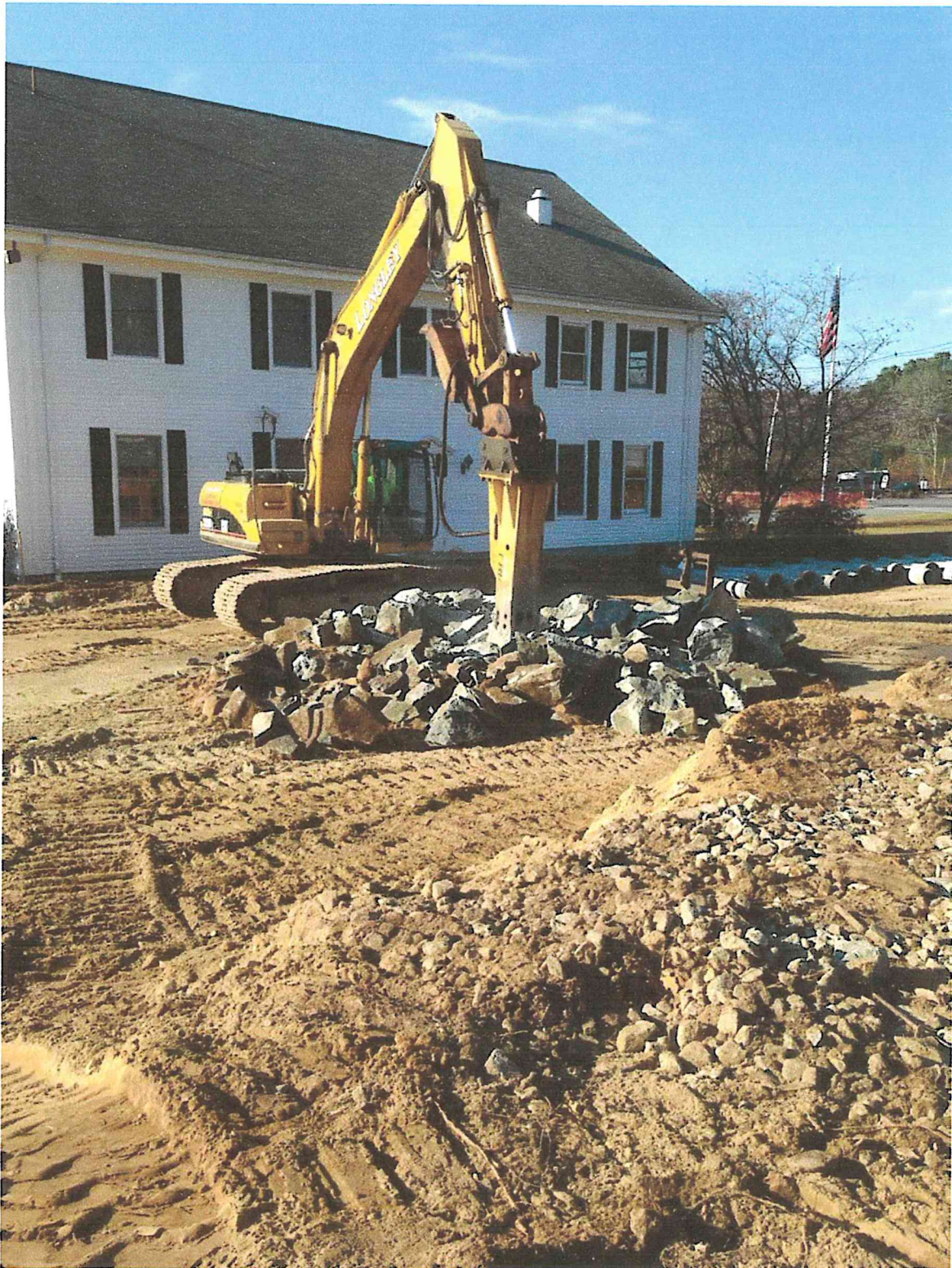
November 12, 2014 – Rock removal using hydraulic hammer adjacent to Fire Station
