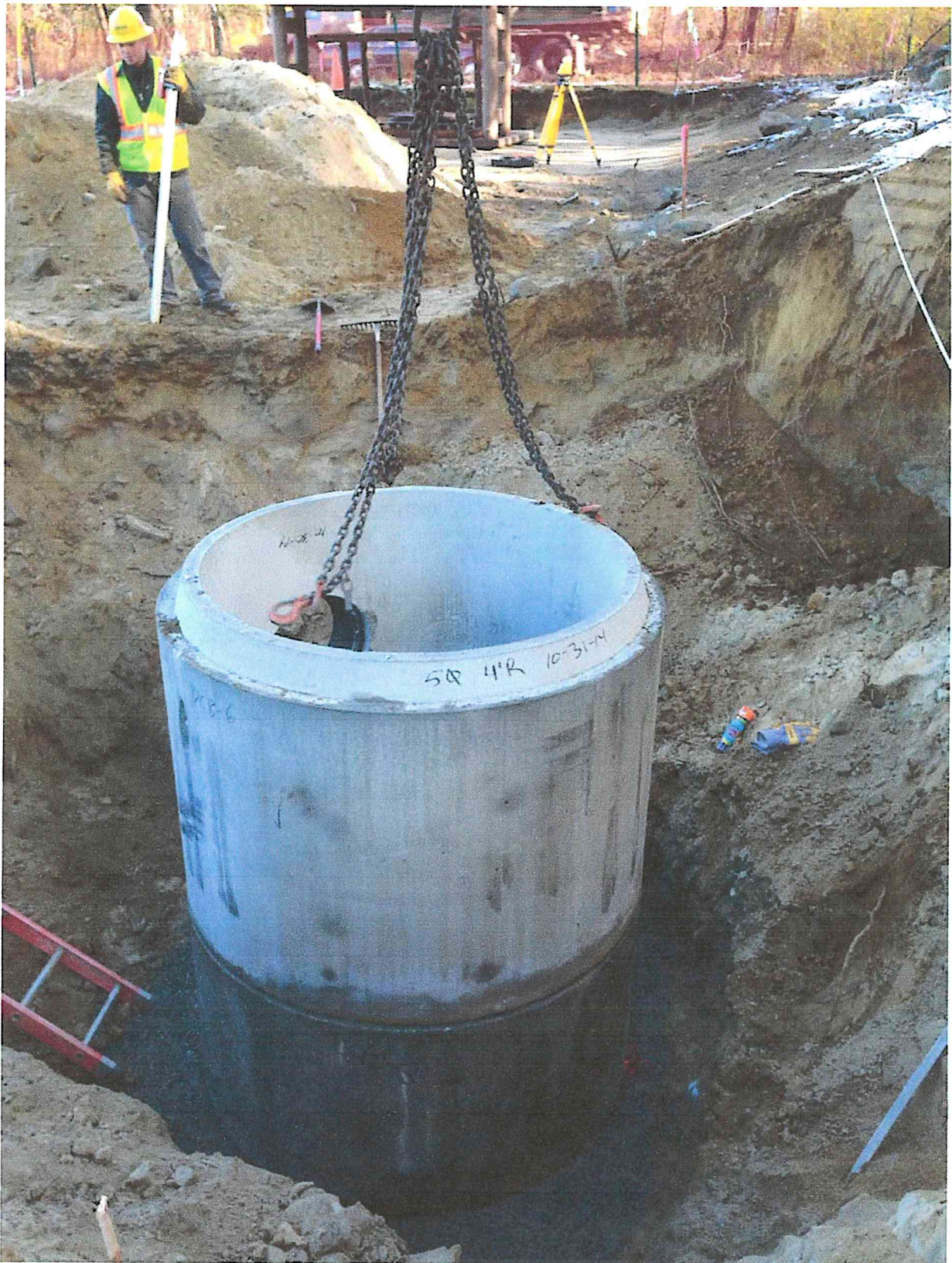
November 14, 2014 – Installation of DCB-6 at Musketahquid Drive
